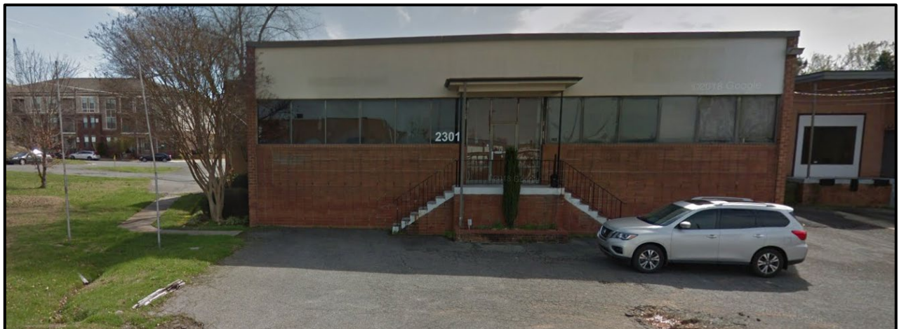
The subject property is developed with a warehouse use.
