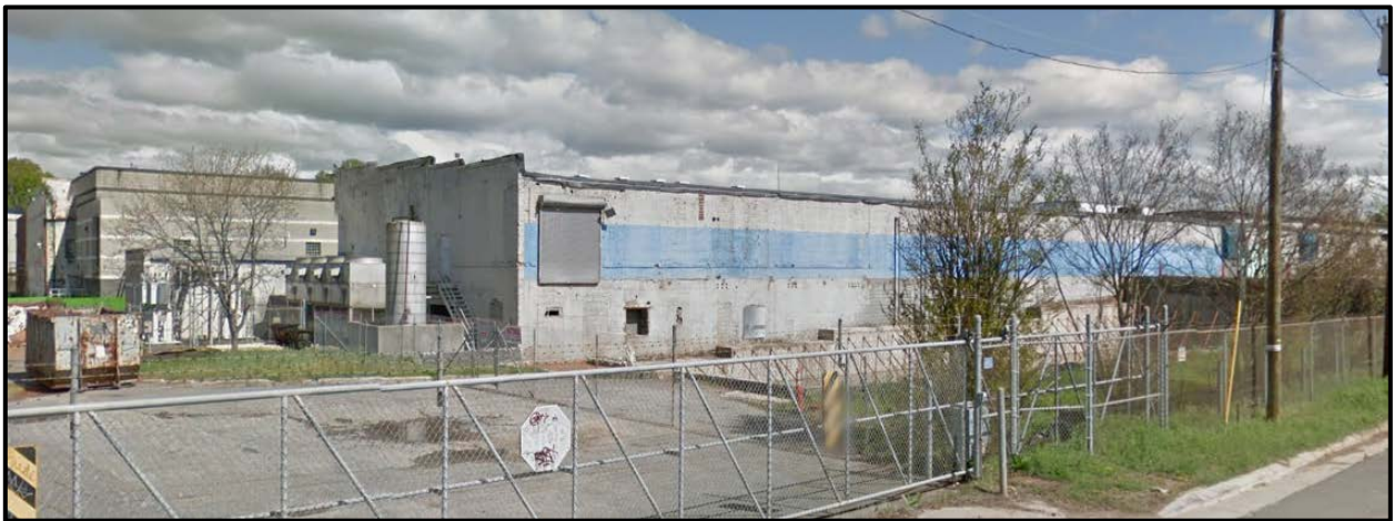
The property to the west along Parkwood Avenue is developed with the historic Highland Mill that is being redeveloped with TOD uses.
