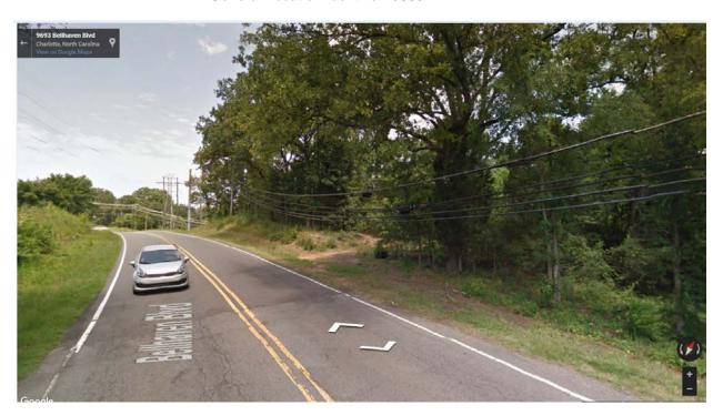
2. CDOT envisions Bellhaven as a three lane section with bike lanes, curb and gutter, planting strip, and sidewalk with maintenance buffer. Half-section is 39' from existing centerline. It is not certain that, as a conventional rezoning, this site would develop this cross section along their frontage and/or provide the necessary right of way/easement.
