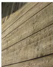
BOARD FORMED CONCRETE
