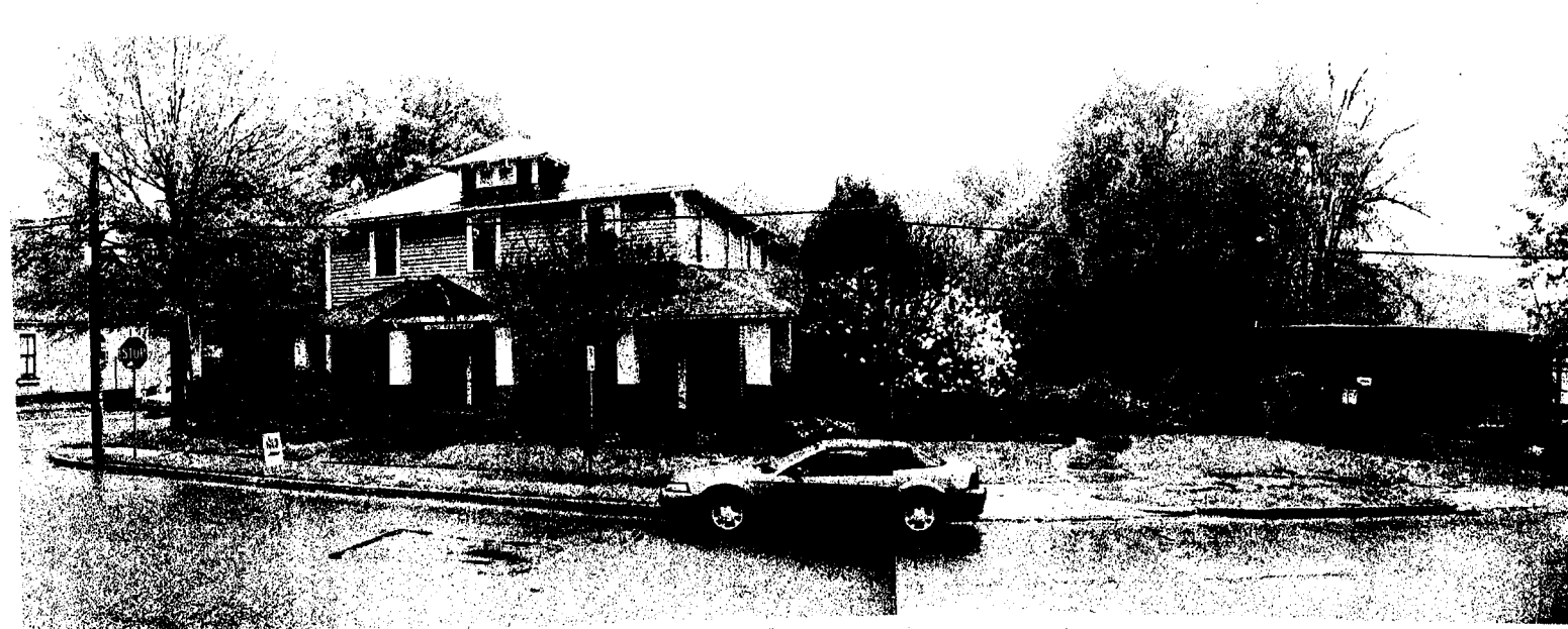
View of the existing building + site along 35 th street.
