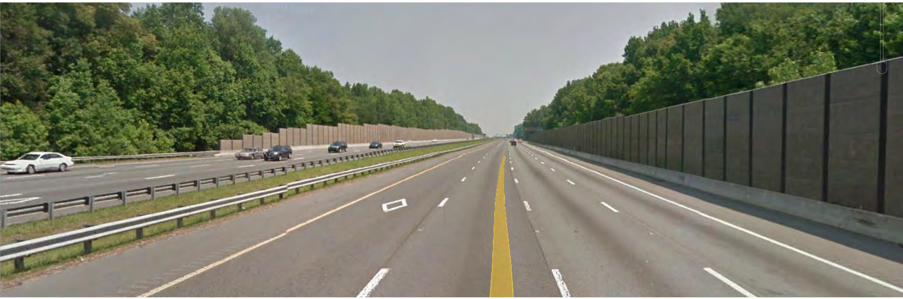
View of I-77 with existing walls
