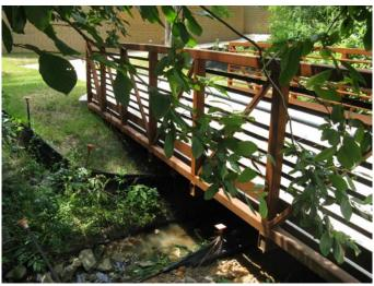
**6A** A bridge is used to connect across the creek, rather than a culvert.
