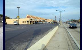
Sidewalks must be a comfortable width (typically 6-10 feet for suburban commercial areas), be separated from the curb with a planter strip of 6-10 feet, be continuous and not open to numerous driveways. In general, the higher the roadway speed the wider the planter strip. This space lacks a sidewalk completely, but even the portion with a walk does not "invite" walking.
