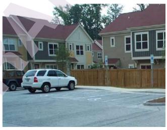
**5C** Six inches of pervious concrete pavement allows surface water to drain through this Wilmore parking lot.
