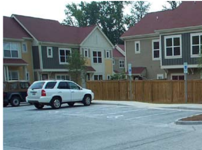
5C Six inches of pervious concrete pavement allows surface water to drain through this Wilmore parking lot.
