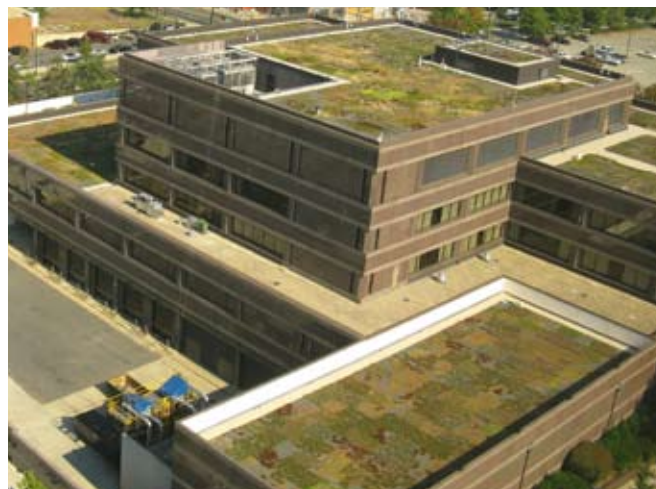
5F Uptown Charlotte's Federal Reserve Bank has a retrofitted green roof that reduces storm water run-off and saves energy.
