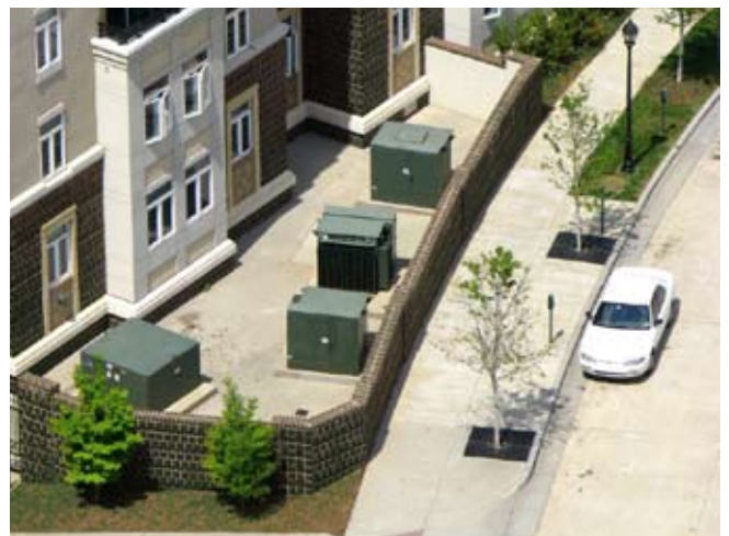
4O A masonry wall incorporated into the building architecture screens these above ground utility structures from view.
