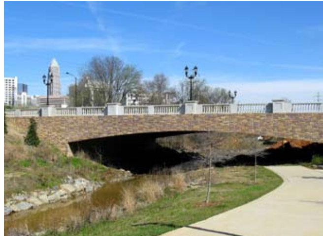
5A Crossing a creek or stream with a bridge, such as this one over Little Sugar Creek, is a better option than a culvert.
