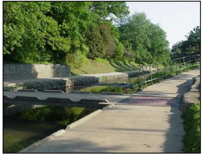
Little Sugar Creek was previously channelized with concrete walls
