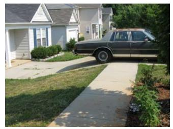
Proper design of driveways ensures parking is accommodated without blocking the sidewalk.
