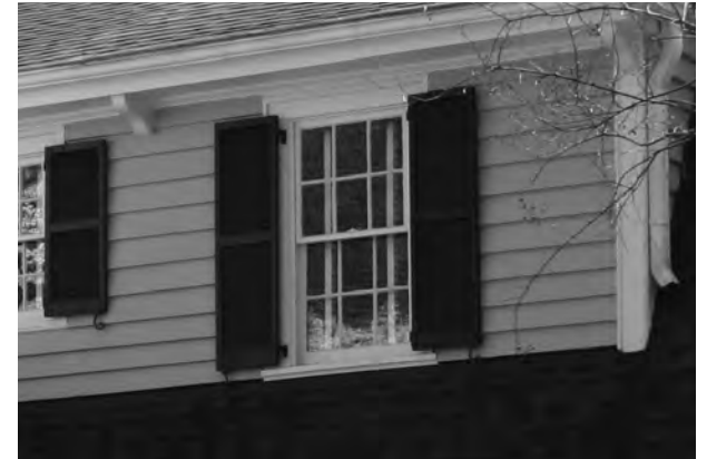
These shutters are properly sized for the window and hung on hinges. When closed the shutters fit the window opening.
