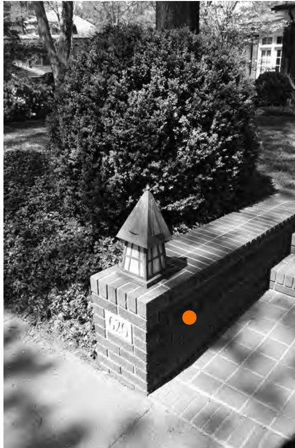
This brick retaining wall defines the edge of the steps and provides an unusual location for a site light fixture. In other instances, a pole mounted fixture would provide illumination for the steps.
