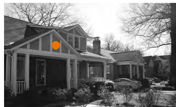
Stucco is often used as secondary material as seen in the bungalow porches above and the Tudor Revival half-timber framing.
