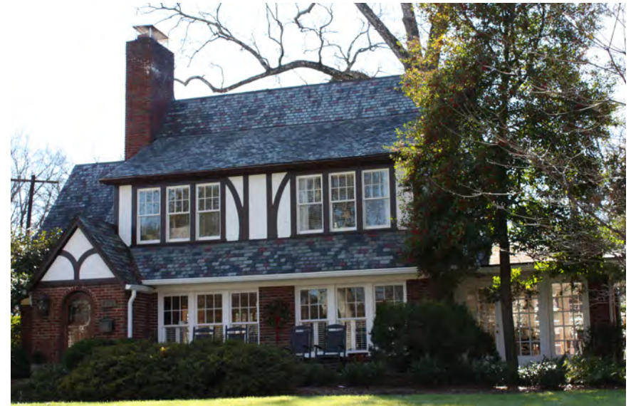
Sets of triple 6-over-1 windows, a massive chimney and half-timber framing are typical elements in this example; note the front terrace, which is seen in several examples throughout the districts as well.
