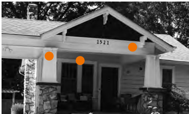
Wood is used for the trim surrounds, columns, eaves, railings and brackets of the two bungalows above.
