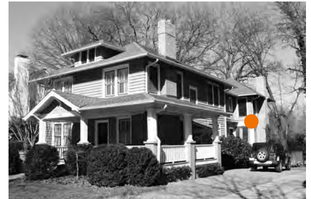
This two-story rear addition, like the example above, respects the vocabulary of the original dwelling with its hip roof, window proportions, and cladding
