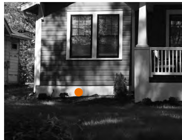
Stucco, like brick, provides a contrasting foundation material on this example.
