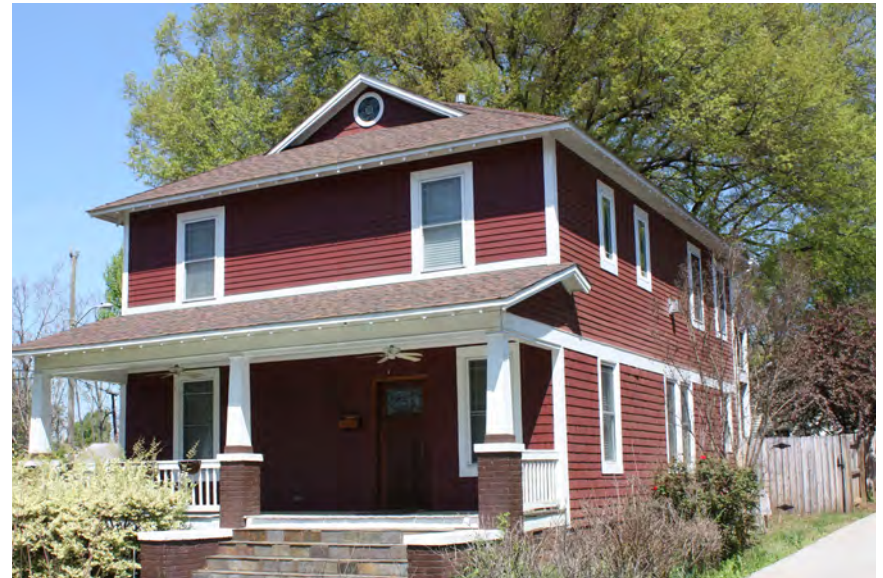
This foursquare has a central roof gable instead of a dormer. The clapboard siding on the first floor is capped by shingles on the second.
