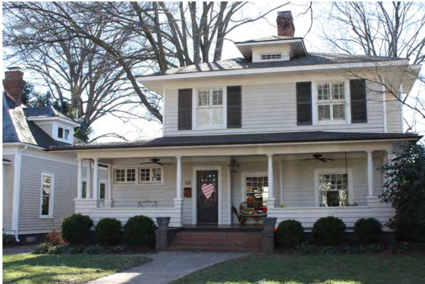
This typical example is characterized by its hip roof, centered dormer, full width porch and side entry door.
