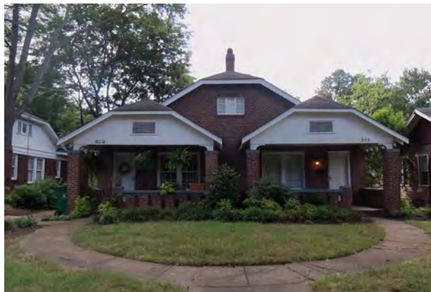
This rare example of a duplex bungalow is unique for its brick cladding and its unusual clipped gable roof forms.
