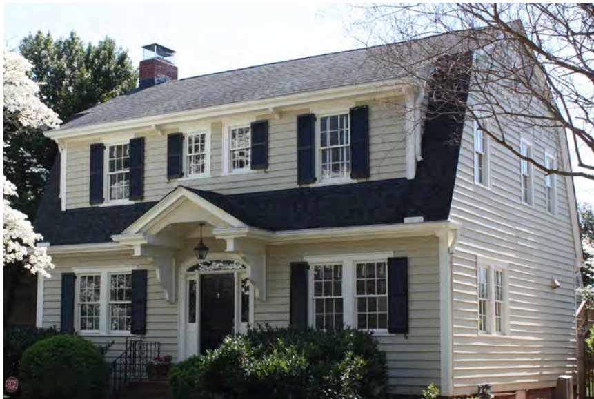
The "Dutch Colonial" is actually a gambrel roof variation. Here the central entry has an elliptical fanlight with sidelights. Paired 6-over-6 windows are typical.
