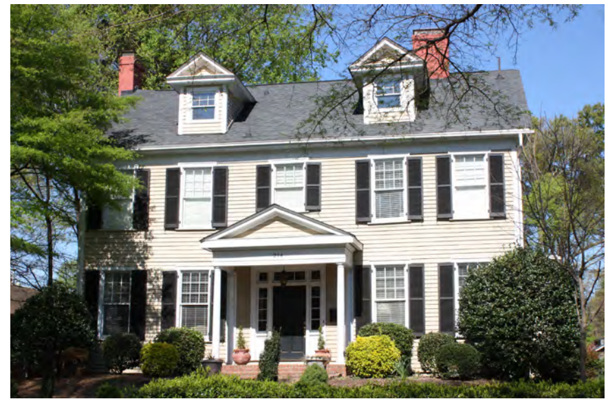
This frame, five-bay, gable-roof, example has roof dormers with pediments that relate to the pediment of the central entrance portico.
