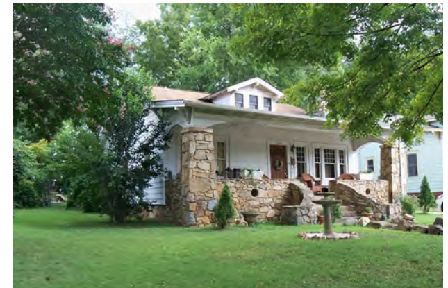
This traditional bungalow has a side gable roof with a shallower pitched section covering the front porch.
