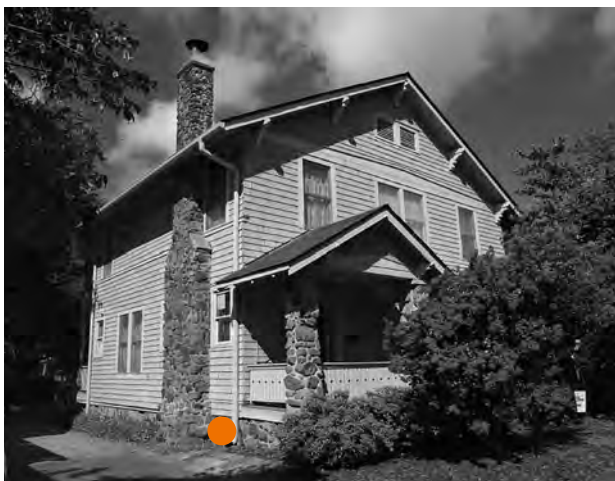
Here, the stone foundation material is also incorporated into the chimney and bases for the porch columns. This technique is commonly found in the districts.
