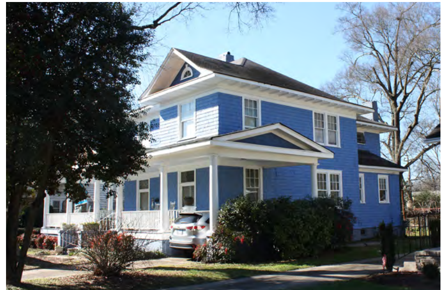
Here, the front porch ends with a gable and extends to create a porte cochere.
