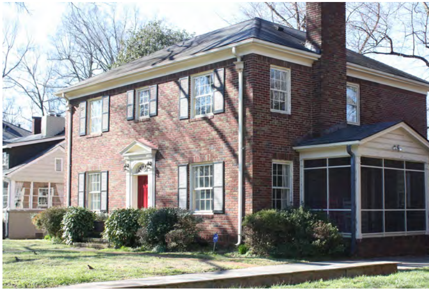
This hip roof, three-bay example has a central entrance capped with a pediment containing a semi-circular fanlight over the door.
