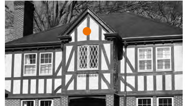
Trim is a significant component in defining styles such as the column and eave details on the bungalow (left) and the flat board trim of the stucco upper story on the Tudor Revival (right).
