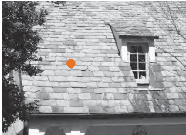
Slate is a distinctive material used on houses throughout the districts. This example is from Hermitage Court.
