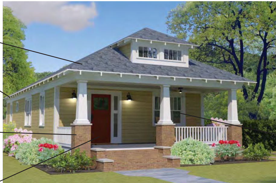
Hipped roof with large hipped dormer
