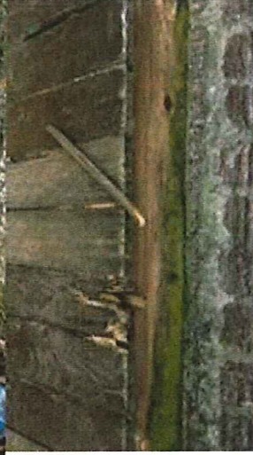
Rotting wood at main entry point
