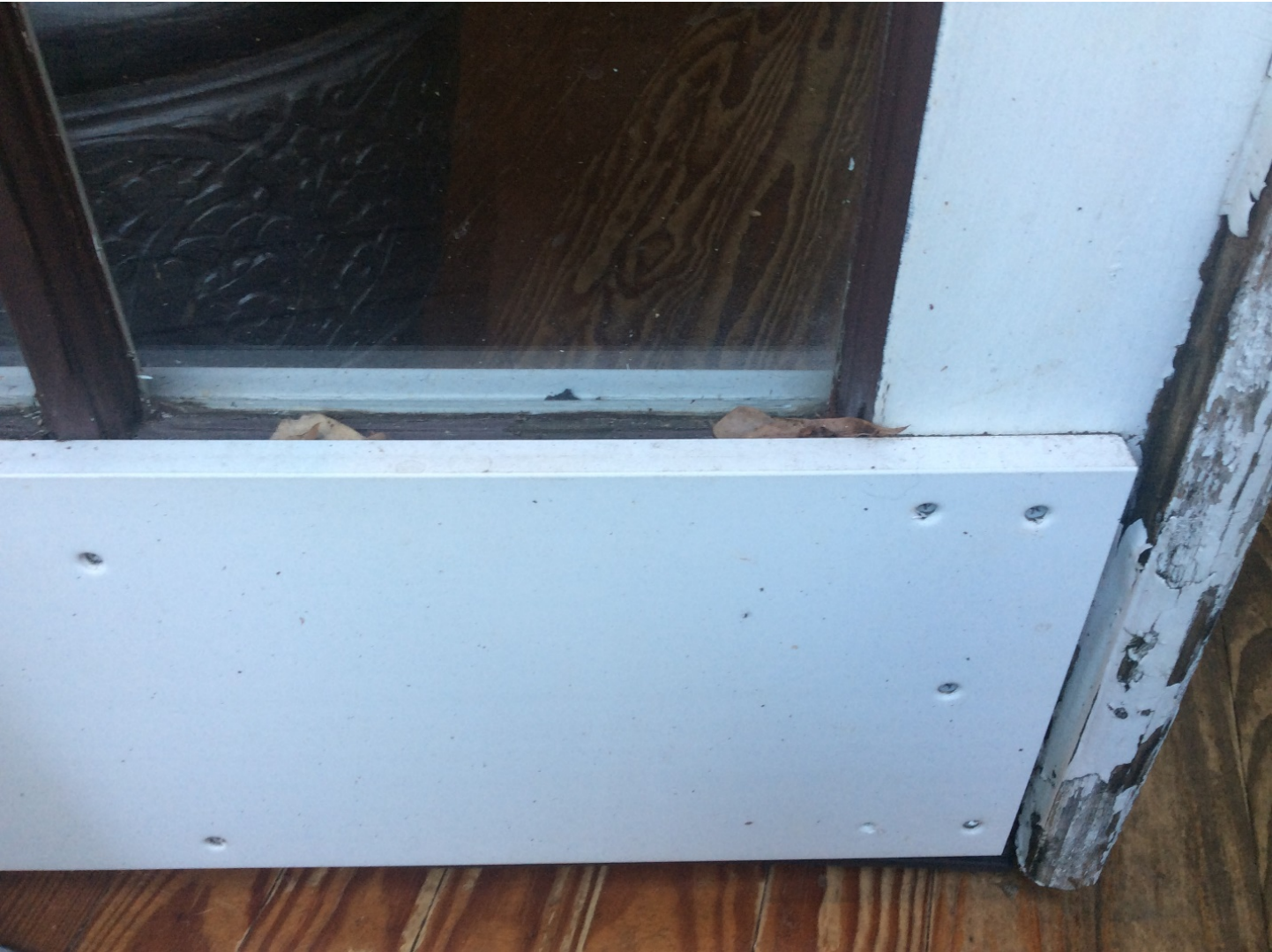
Nailed in board to stop more water
