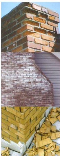
Severe spalling and deterioration is caused by water penetration.
