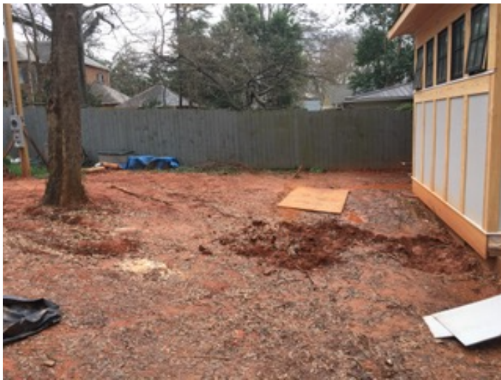
Back yard of property. Current tree elevation per survey 721 ft, back of house elevation 719.8ft . Grading away from house will require per code an addition 6% for 10'.
