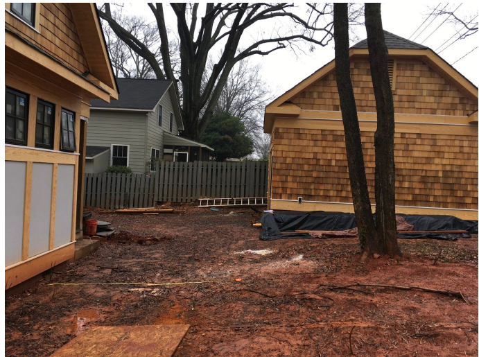
Tape indicates 10ft from rear of house, tree is 18ft. Note tree elevation to rear of house before grading per code. Root system will be significantly jeopardized and any mitigation will not support long term sustainability.
