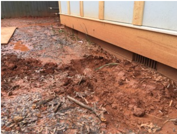
Current back of house elevation, in addition to code, grading needed for Drainage away from house.
