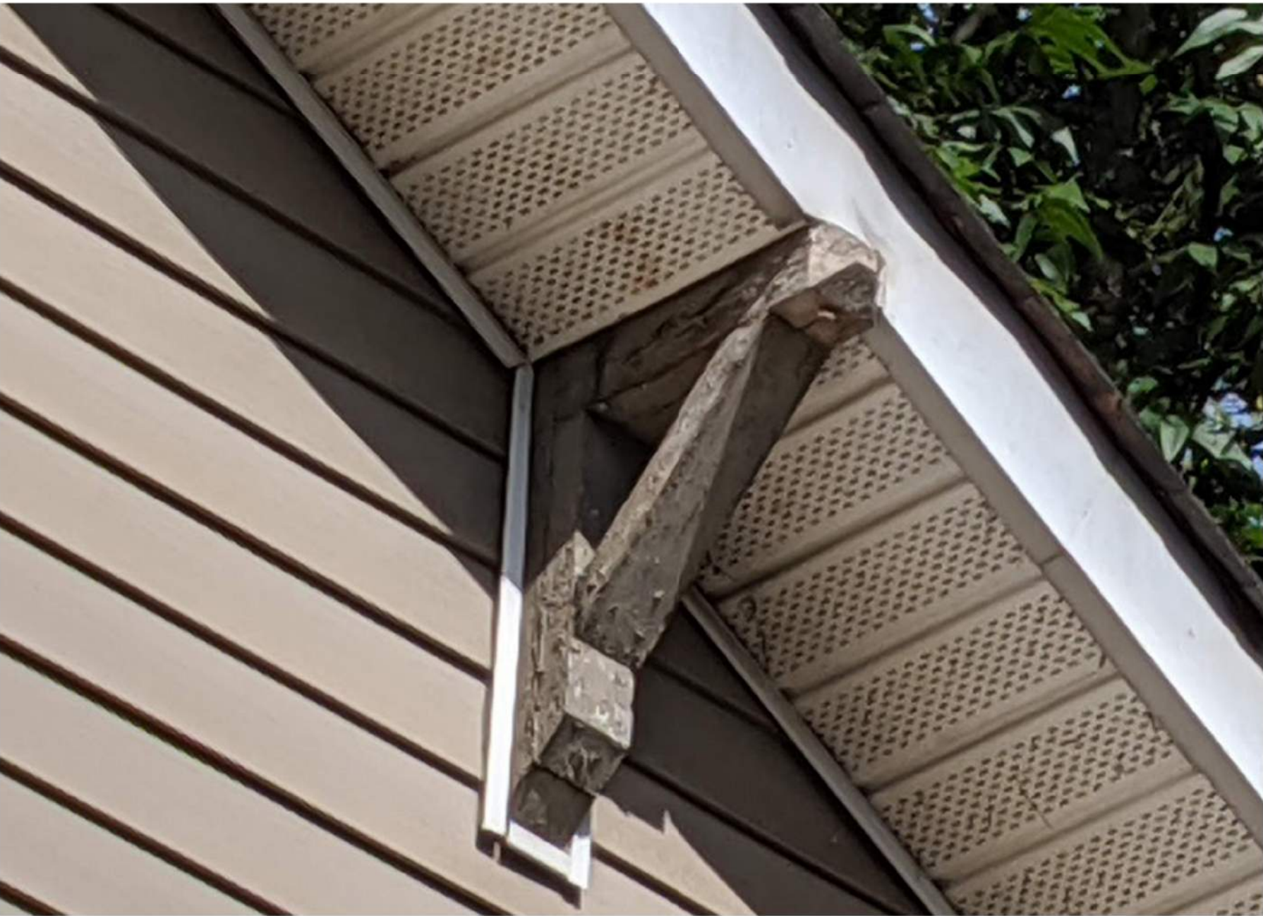
Existing Roof Bracket on Accessory Building
