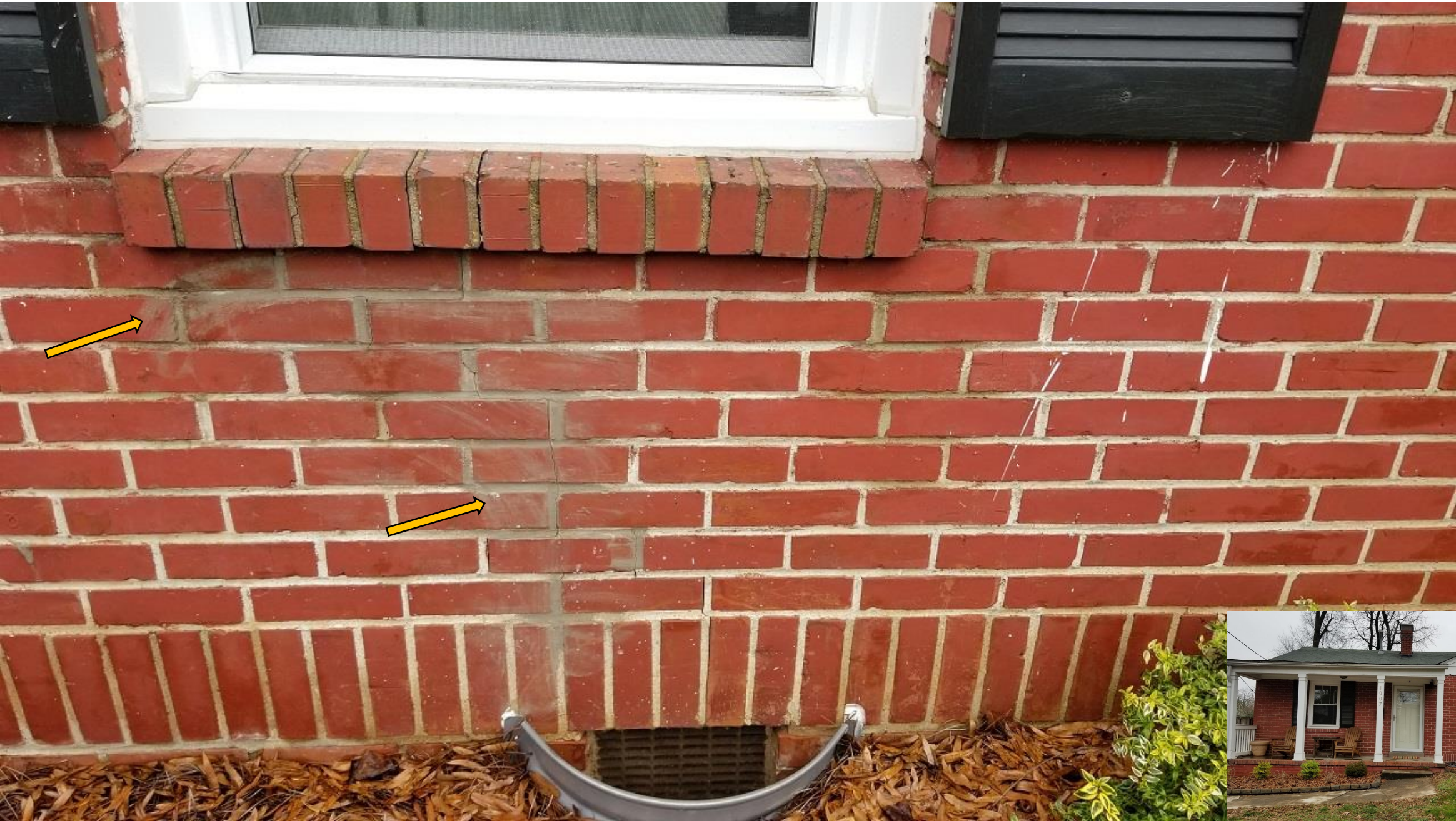
Closer view of some of the repair work. No apparent attempt made to color or blend with the rest of the house.
