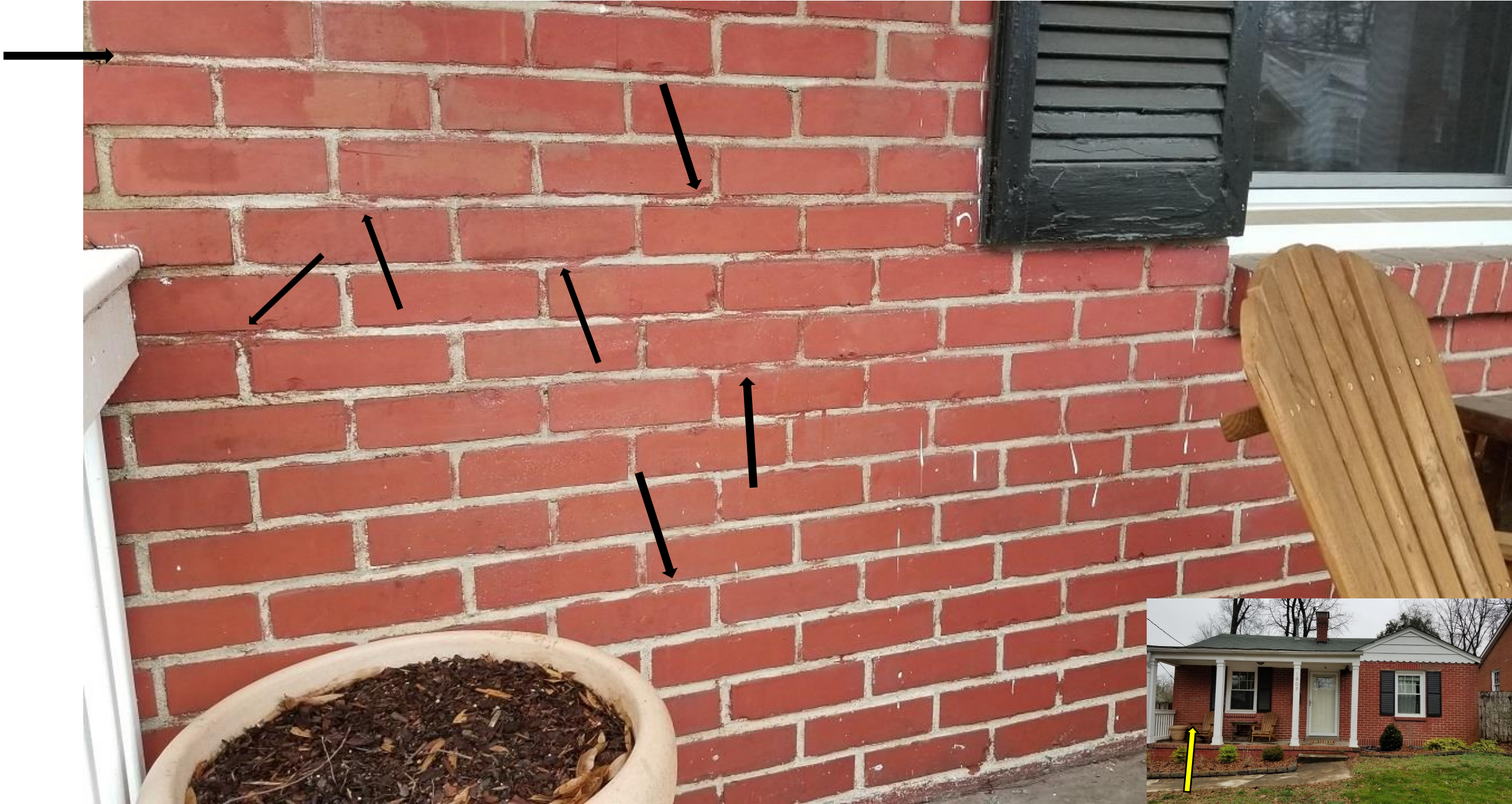
Examples of rather sloppy painting coloring the mortar. White paint drips are either from painting the mortar or other painters doing the trim.
