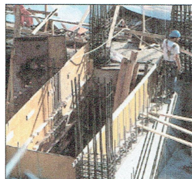
HDO panels can be reused many times in concrete forming.
