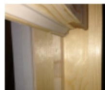
Side Jamb detail with Hidden Balance
