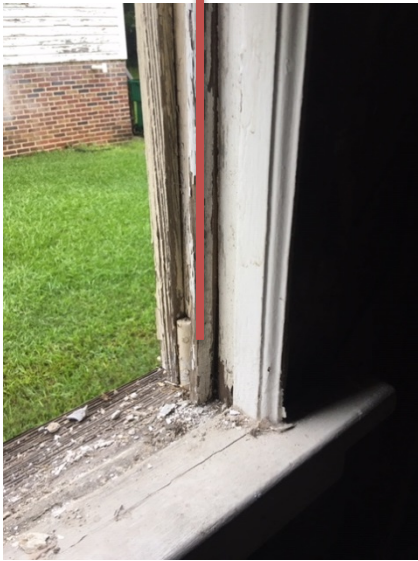
Excessive rot and detachment
