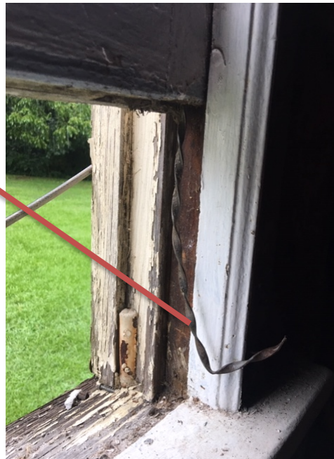
Spiral rod balance system compromised
