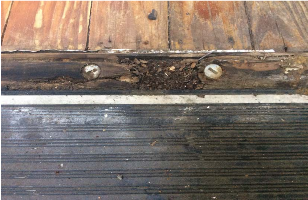
Rotted deck/door threshold
