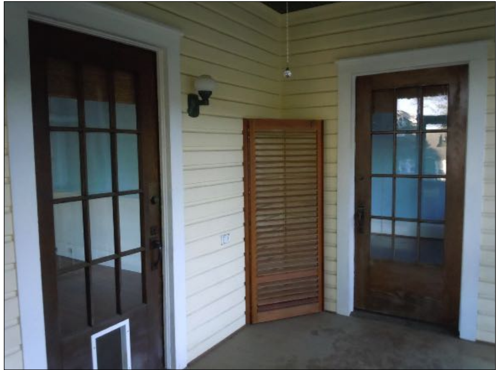
DOOR OPENINGS TO REMAIN COMPROMISED DOORS TO BE REPLACED
