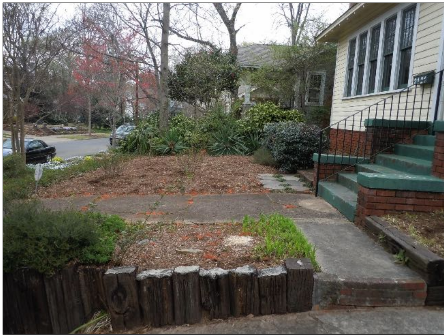
FRONT YARD RETAINING TO BE REPLACE WITH CURB AND RECESSED PLANTER AS RETAINING & CRACKED CONNECTING CONCRETE WALK TO BE REPLACED WITH NEW & A BRICK BORDER TO BE ADDED
