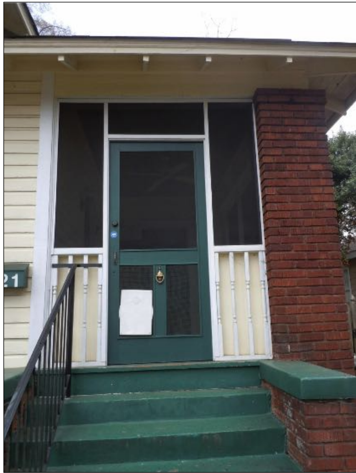
FRONT PORCH REMOVE SCREEN, OPEN FRONT PORCH GREEN PAINT TO BE REMOVED
