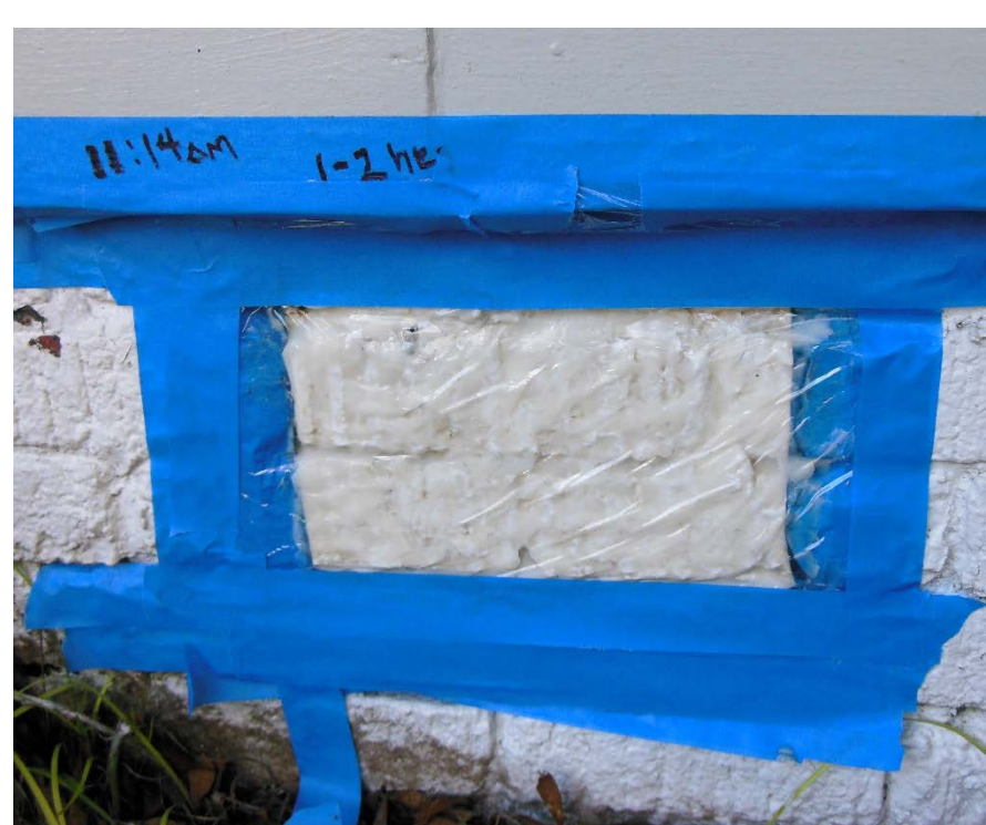
Paint Striper Re-Applied & Insulated
