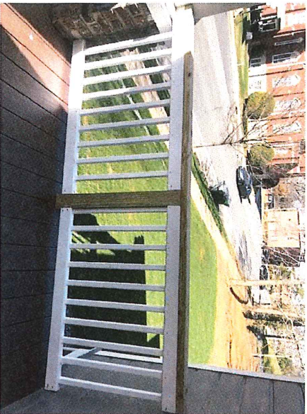
Flip Railing around. Smooth side to face the street.
