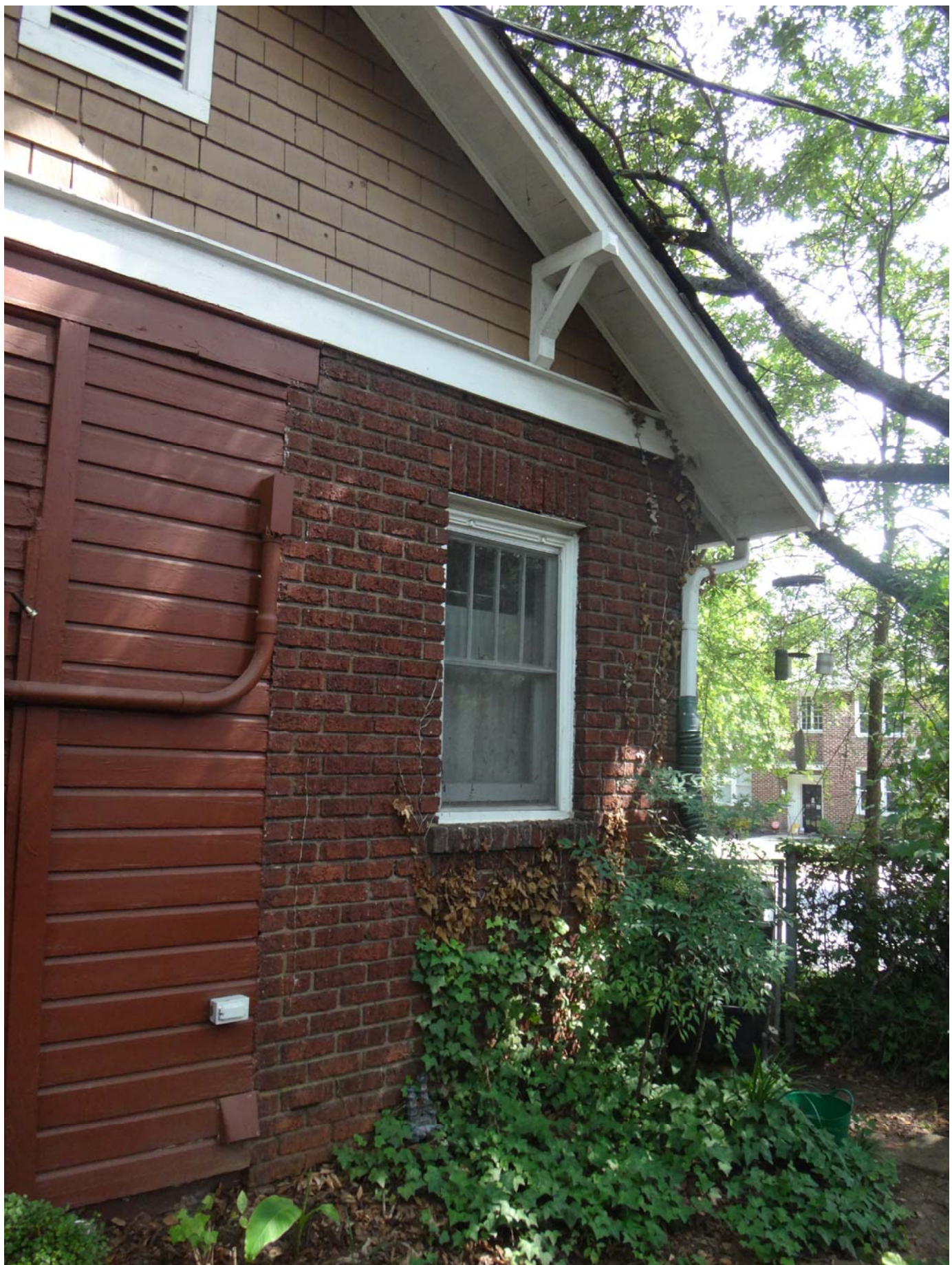
DETAILS - SHINGLE, DUTCH LAP, BRICK, BRACKETS, RAKE & EAVE, WINDOWS
