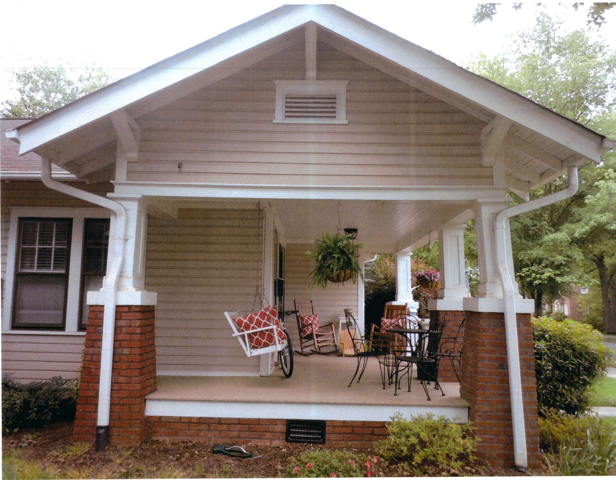
THE FAR LEFT FRONT BRICK PIER IS OFF PLUMB. IT WILL BE STABILIZED WITH HELICAL PIERS AND /OR PRESSURE GROUTING.
