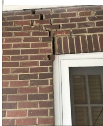
Settling over side porch entry door
