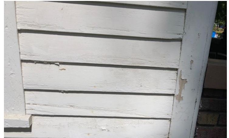
Existing Wood Siding to be repaired and Repainted
