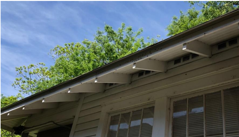
Existing Eave Detail to be replicated on Addition
