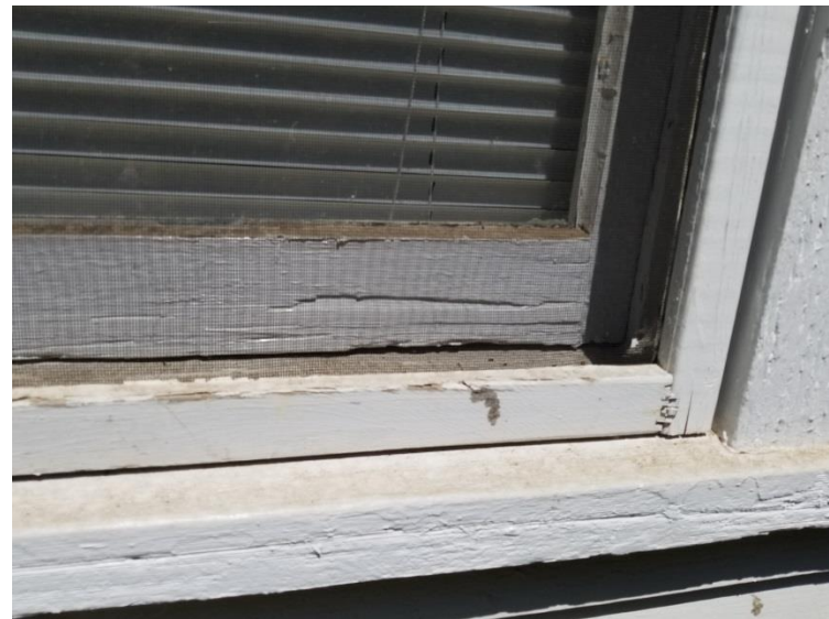
Sashes in bad condition and screens missing or damaged
