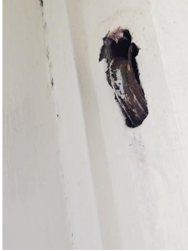
Most balances are missing
