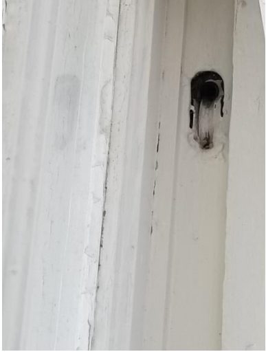
Most balances are missing
