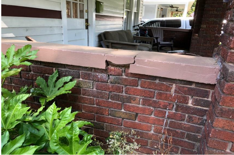
Condition of Existing Brick Rail
