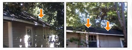
**SUMMARY** Multiple nail pops were noted throughout the entire roof that need to be corrected properly to prevent the nail from damaging the shingle and/or allowing possible wind and/or water damage.
