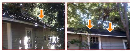
4. Multiple nail pops were noted throughout the entire roof that need to be corrected properly to prevent the nail from damaging the shingle and/or allowing possible wind and/or water damage.
