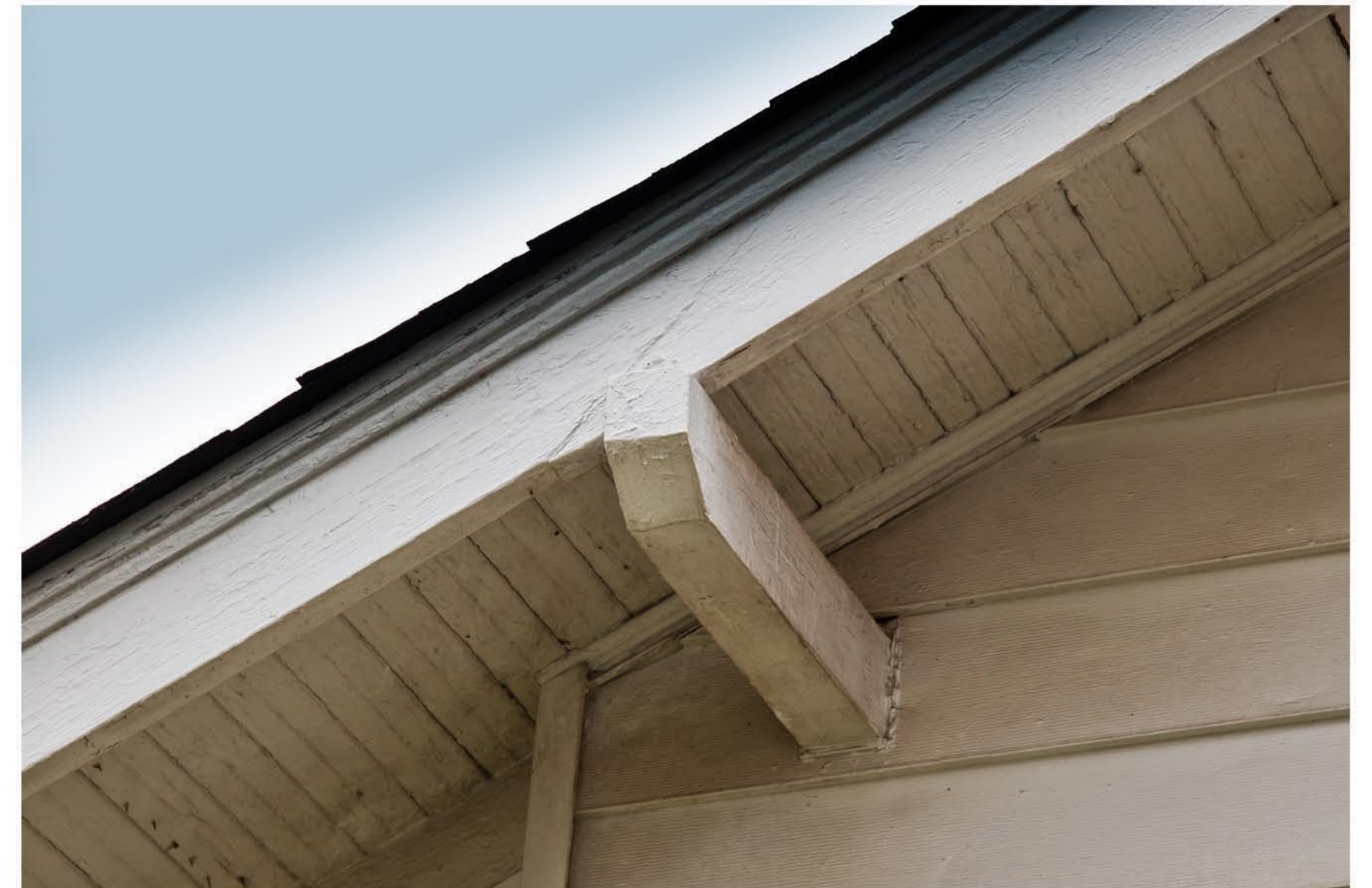
Detail - rafter bracket
