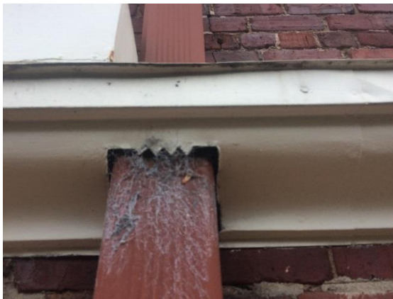
Downspouts are cut through the banding at various levels making them difficult to maintain. Birds and other animals can build nests and gain access to the cornice detail.
