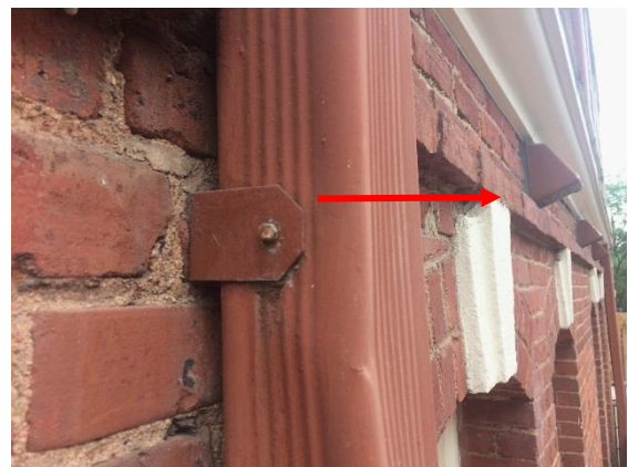
The downspouts are painted to match the brick color and the current material is not "historic". These downspouts are typical of what homeowners purchase and install today.
