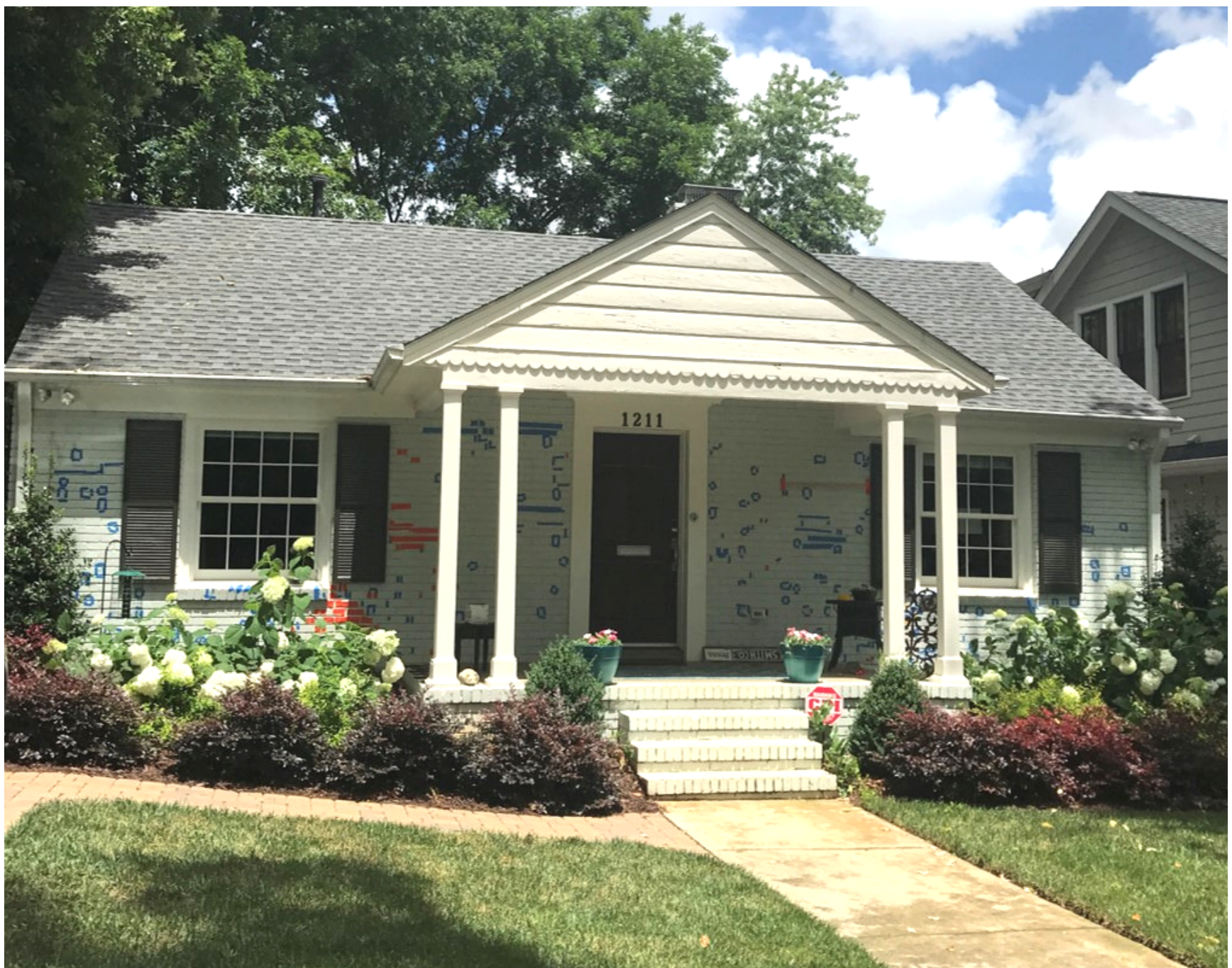
Blue and orange tape signifies brick, joint, and mortar irregularities
