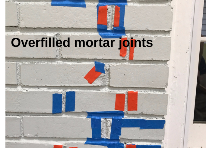
Overfilled mortar joints and cracking
