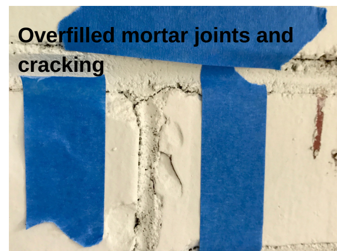
Inconsistent mortar joint width
