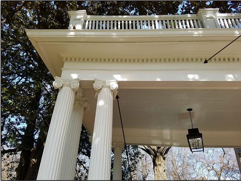
Column detail to match existing home
