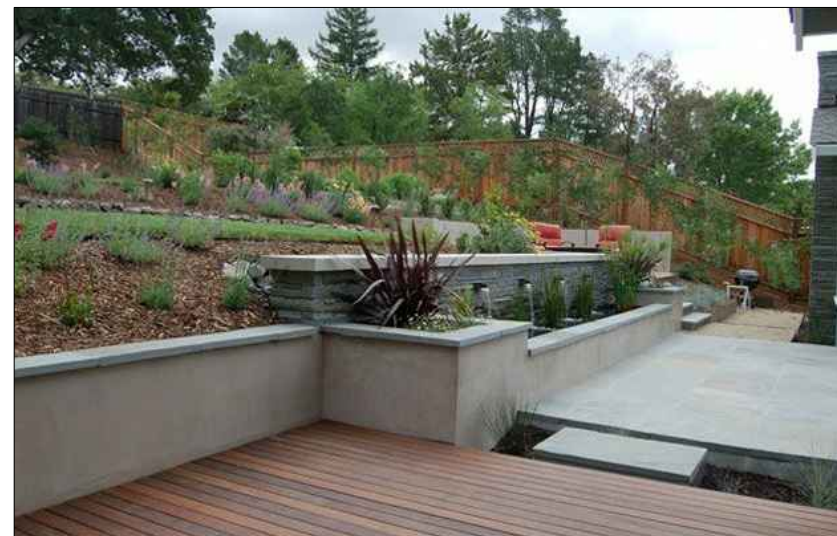
STUCCOED RETAINING WALLS W/ BLUESTONE CAPS
