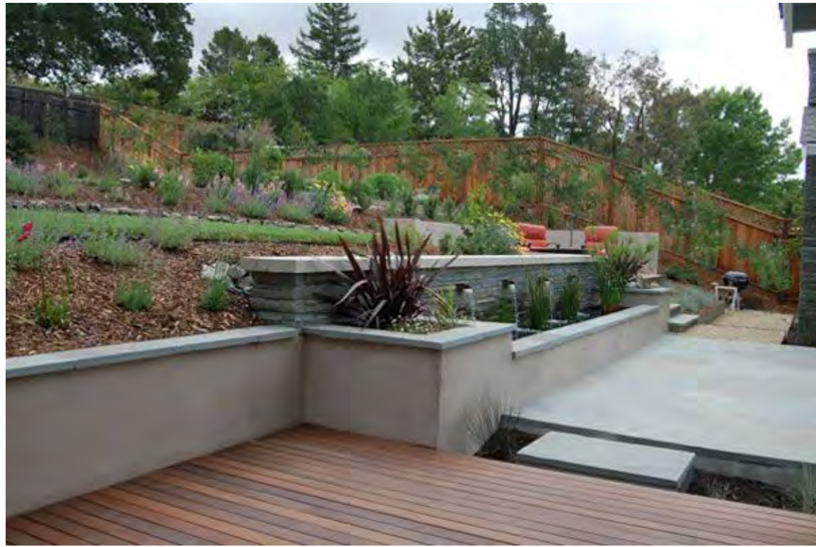
STUCCO RETAINING WALL WITH STONE CAP
