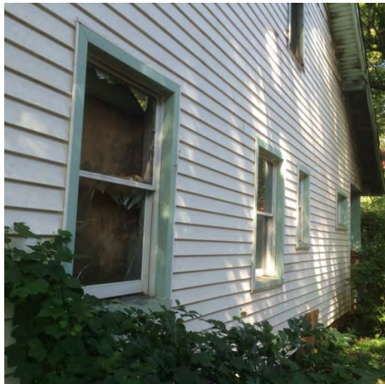
BELOW:: Left of house showing melted/charred siding, broken windows, and demolished 2 nd floor & roof. Damage goes from rear to front, top to bottom.
