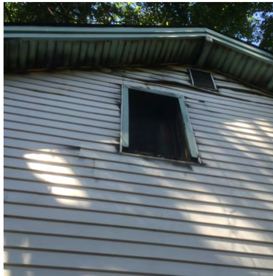
BELOW:: Left of house showing melted/charred siding, broken windows, and demolished 2 nd floor & roof. Damage goes from rear to front, top to bottom.
