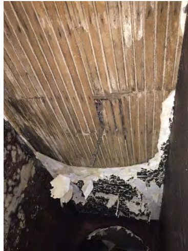
ABOVE: Indoor Ceiling showing melted coverings, mold, axe and water damage. Unsalvageable.
