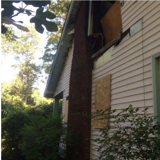
ABOVE: Right side of house showing unsalvageable melted/charred siding, broken windows and demolished 2 nd floor & roof
