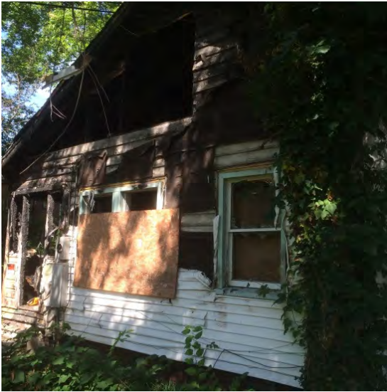
ABOVE: Rear/Left of house showing melted/charred siding, broken windows, and demolished 2 nd floor & roof
