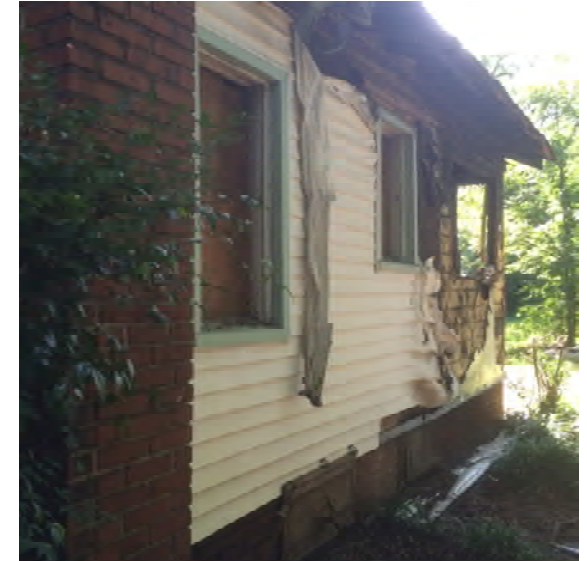
ABOVE: Right side of house showing unsalvageable melted/charred siding, broken windows and demolished 2 nd floor & roof
