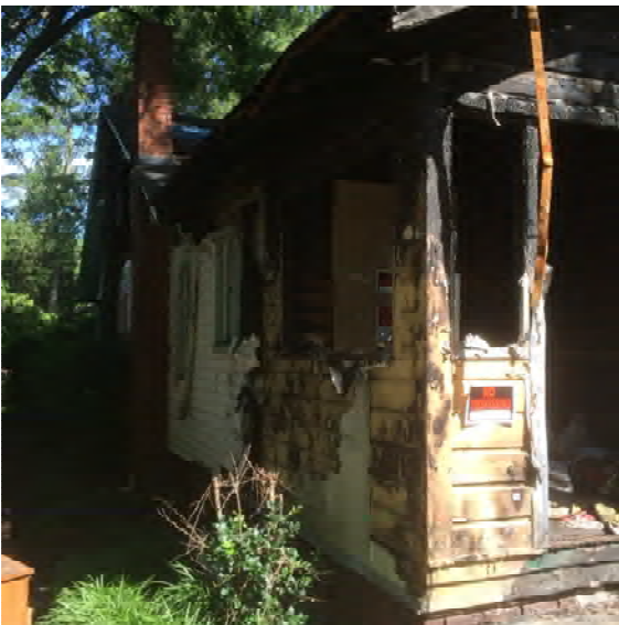
BELOW: Rear including Roof and Kitchen area. Unsalvageable structure from top to bottom.
