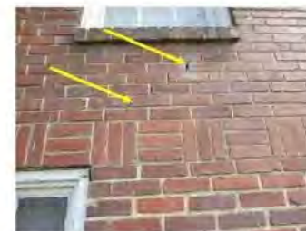
Cracks in the brick veneer were observed on the left, right, and rear sides of the house.
