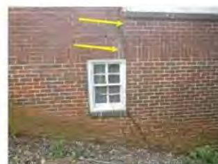
The cracks in the brick near the right rear corner
