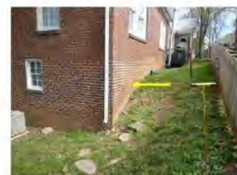
The wall is bowing inward
