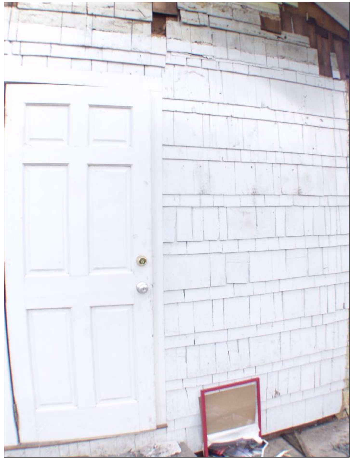
SHOWING INTERIOR WALL (SHAKES) OF SHED ADDITION BUILT IN 80'S-90'S AT (SOUTH REAR) OF HOUSE
