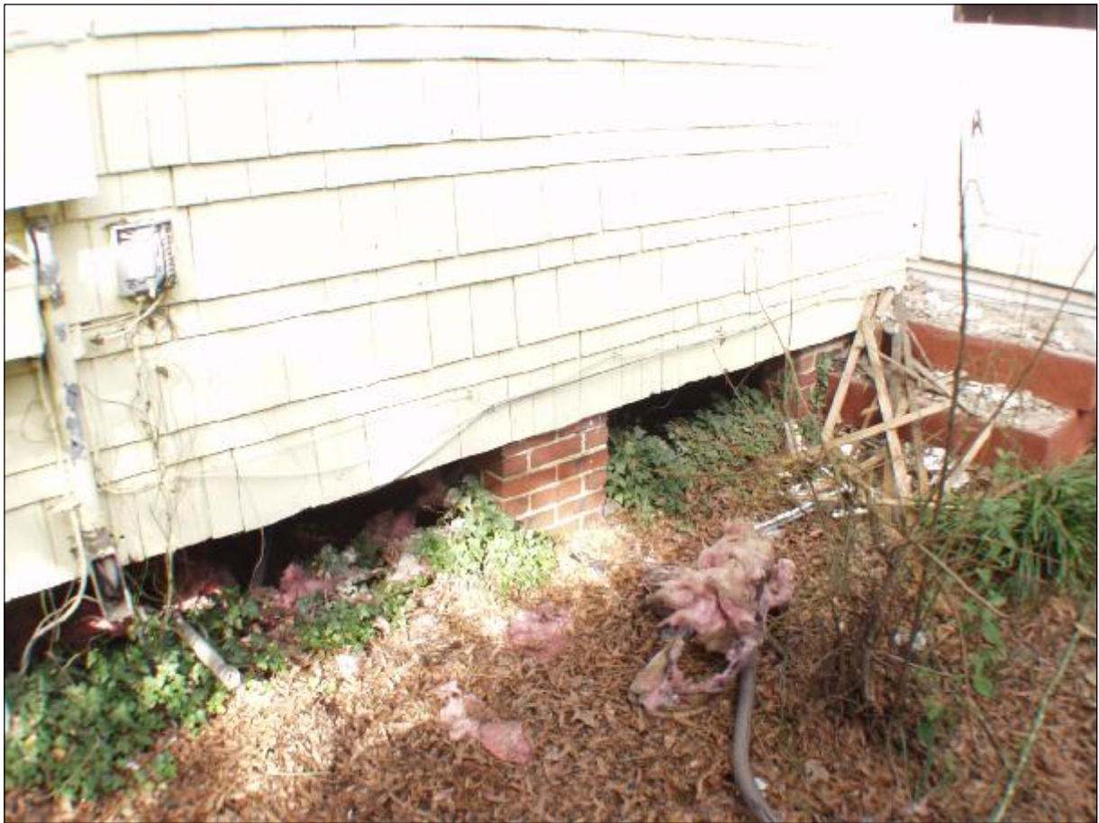
AREA OPEN UNDERNEATH PAST ADDITION
