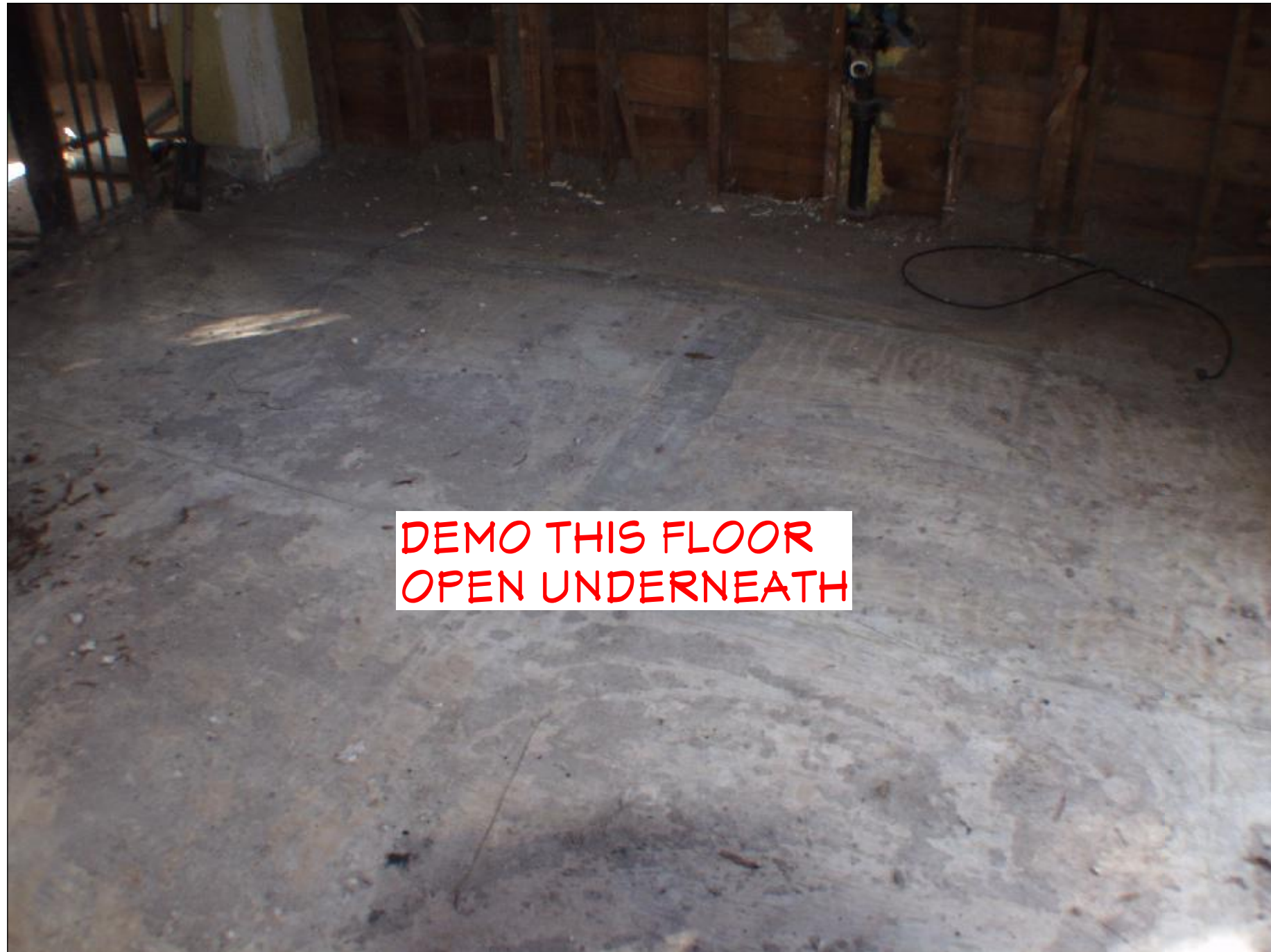
SHOWING PLYWOOD FLOOR IN AREA OF CONVERTED PORCH (WEST REAR)
