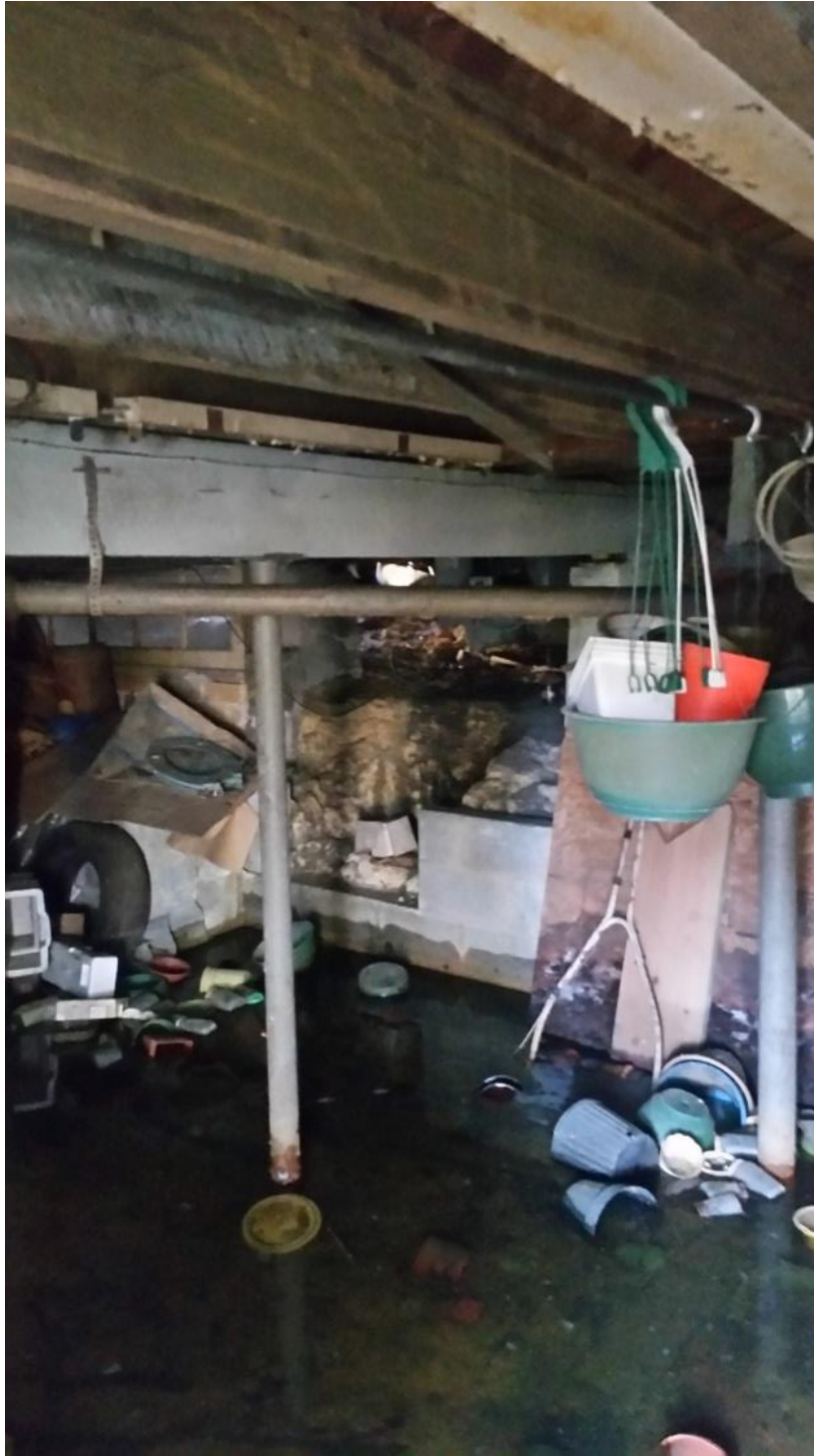
Standing Water in the Crawl Space
