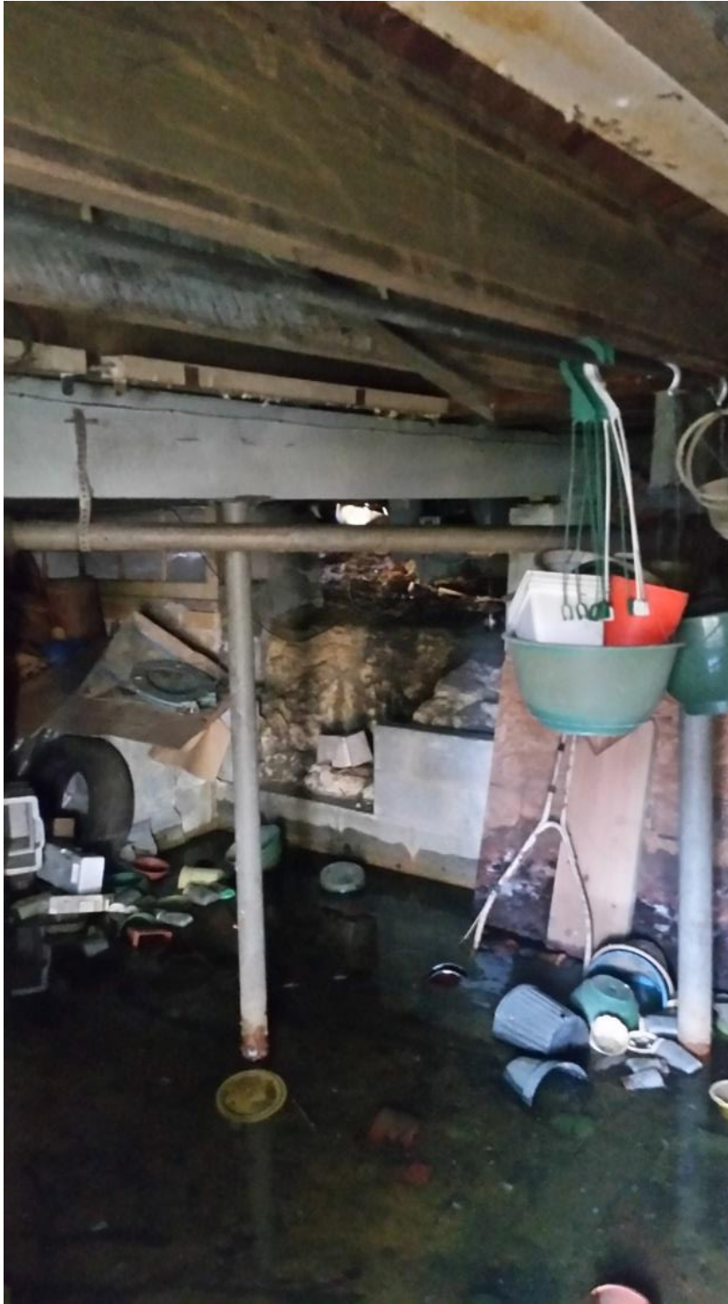
Standing Water in the Crawl Space
