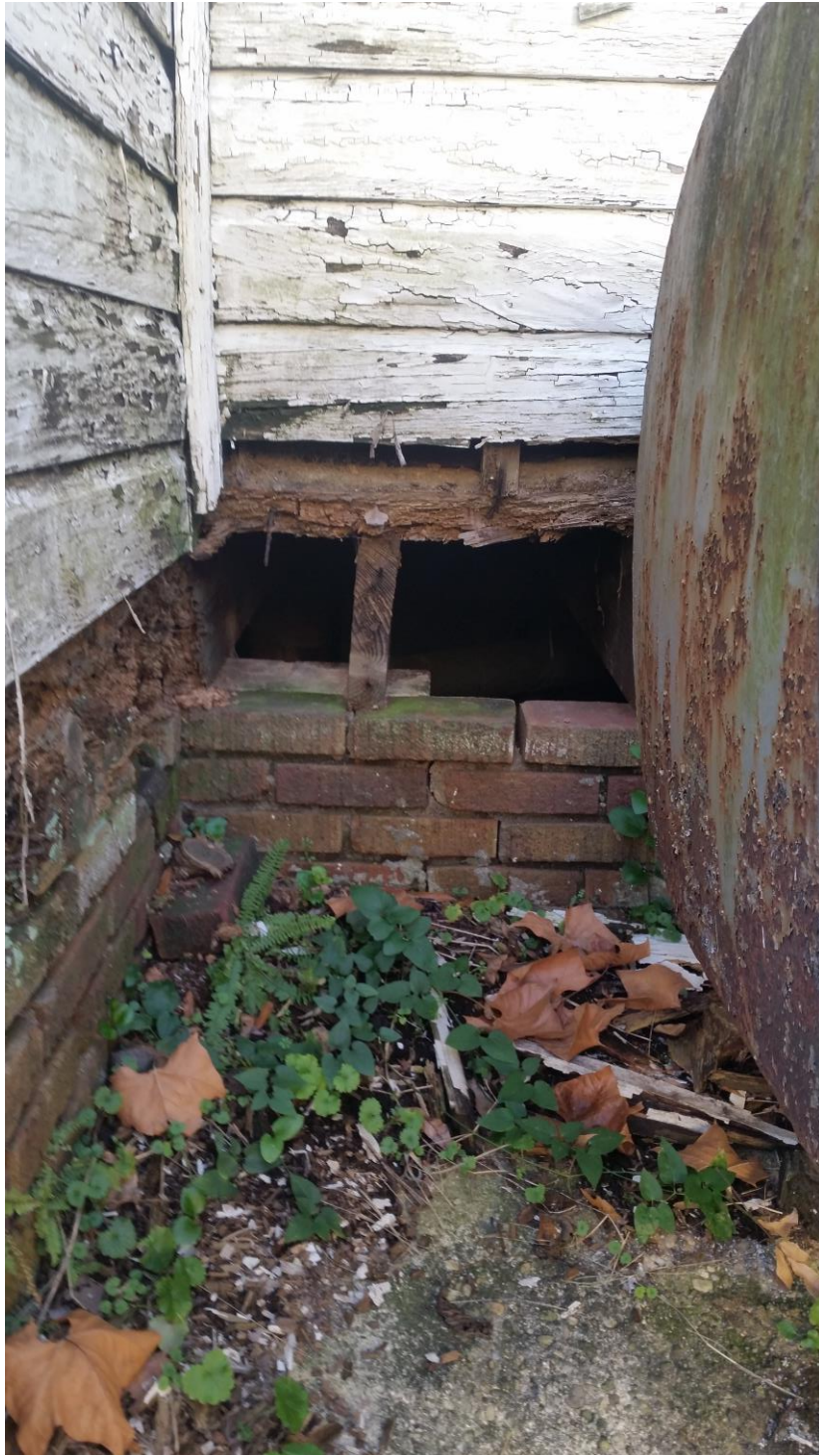
Compromised Foundation and Structure
