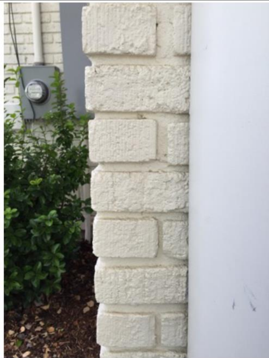
Left wall of 2006 rear porch addition. Vastly inconsistent mortar head (vertical) joints, ranging from 1" at top to 3/8" at bottom. Bed joints also vary as well. Also note broken and crooked bricks, and excess mortar on brick faces & edges.
