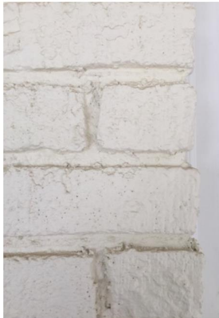
Shoddy brick & mortar installation, left wall of 2006 addition
