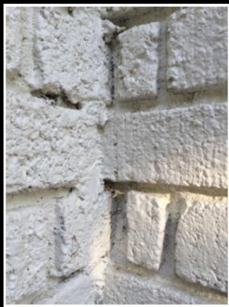
More inferior, shoddy brick & mortar work- SW side butt joint of '06 addition & orig. bldg.
