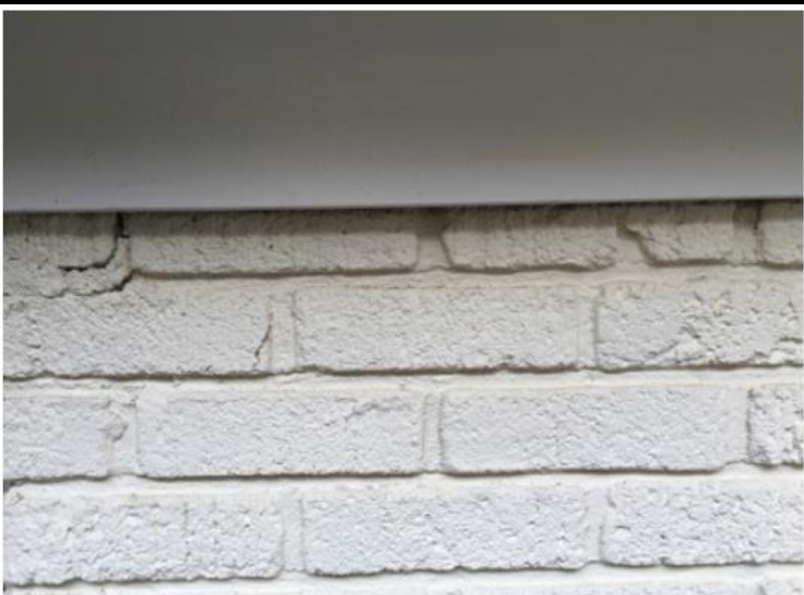
Broken bricks, uneven mortar spaces, sloppy mortar finish. Top of 2006 addition SW wall (facing Worthington Ave)
