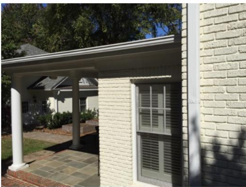
Inferior brick and mortar work on South wall of '06 addition (w/window) hidden by paint. Disparate elements of garage, addition and original house unified with neutral color.
