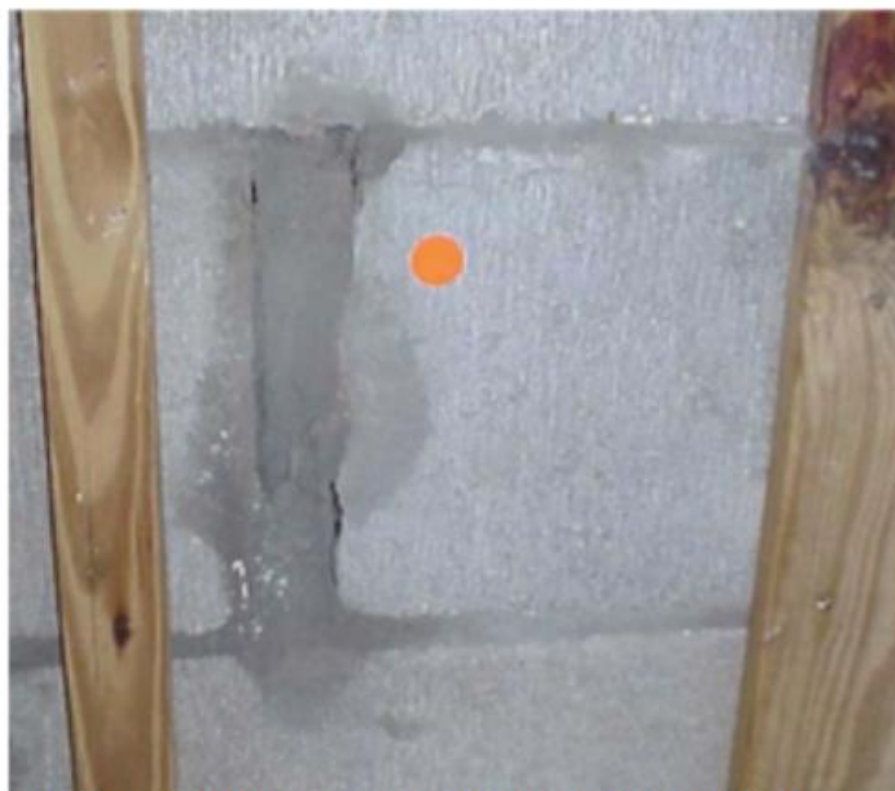
FIGURE 2: Improper mortar joint thickness.
