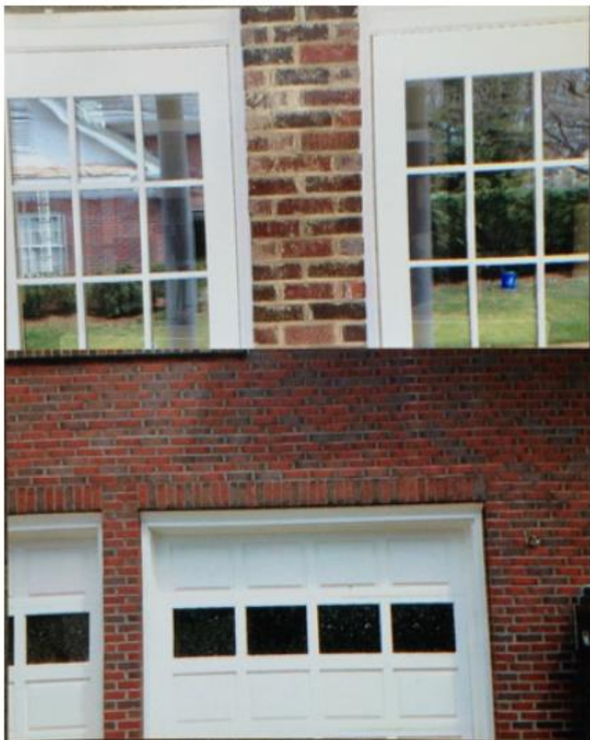
Photos of mismatched brick & mortar colors, between house (top) and garage (bottom). Also note mismatch in reflection on left side of top photo.
