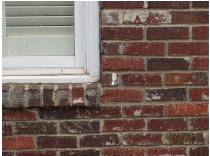
More sloppy, unsightly masonry work— north side wall of 2006 addition.
