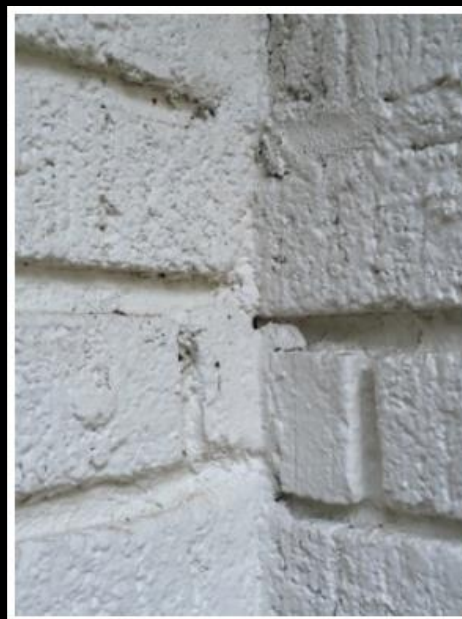
More inferior, shoddy brick & mortar work- SW side butt joint of '06 addition & orig. bldg.
