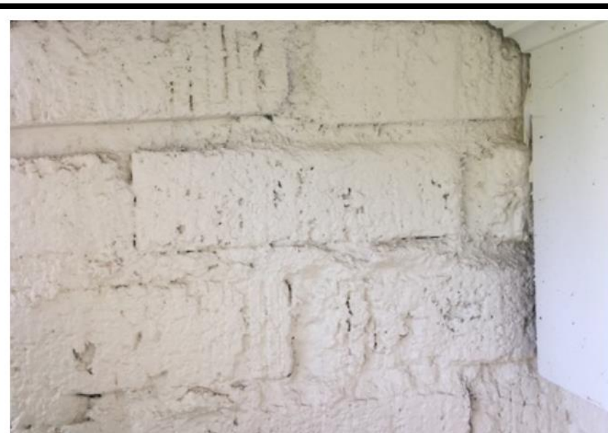
Shoddy and overfilled mortar joints, upper NW wall of 2006 addition
