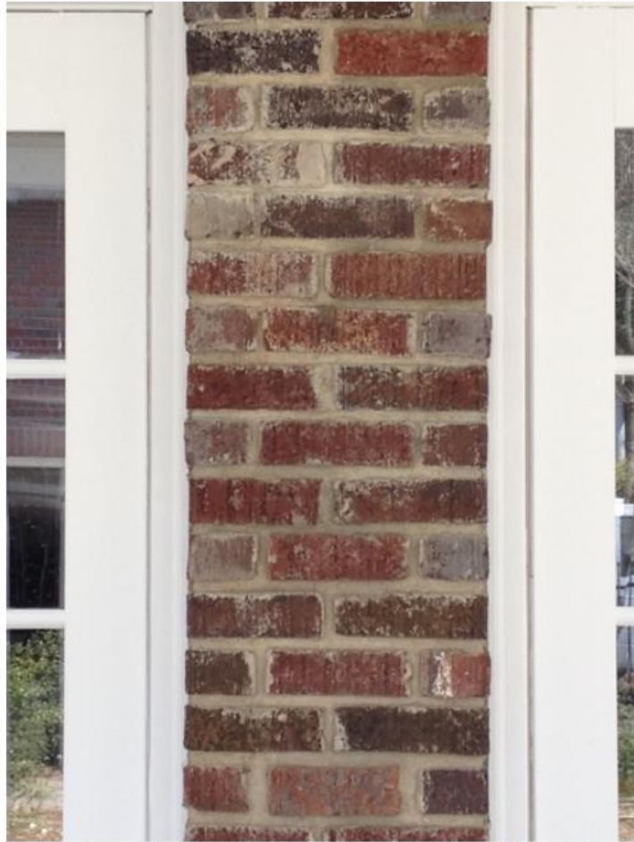
Further evidence of poor quality masonry installation- center wall of porch addition. Note the crooked bricks, excess mortar and inconsistent joint spaces. Also note the mismatched red and gray garage brick in the left reflection.
