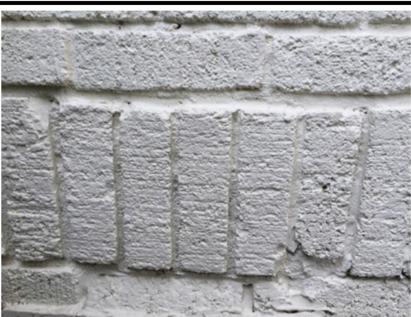
More NW wall with crooked, protruding soldier course and caved-in brick below.
