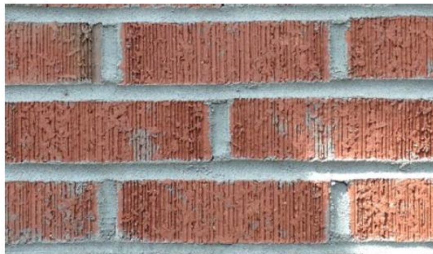
Mismatched brick texture and brick & mortar colors, between the 1924 house (top) and 2001 garage (bottom)
