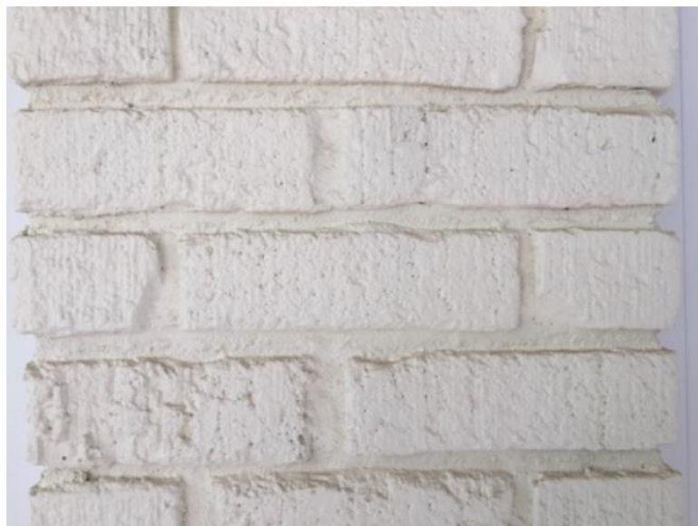
Inconsistent mortar joint widths; crooked and broken bricks; sloppy & excess mortar. Center wall of 2006 rear porch addition.
