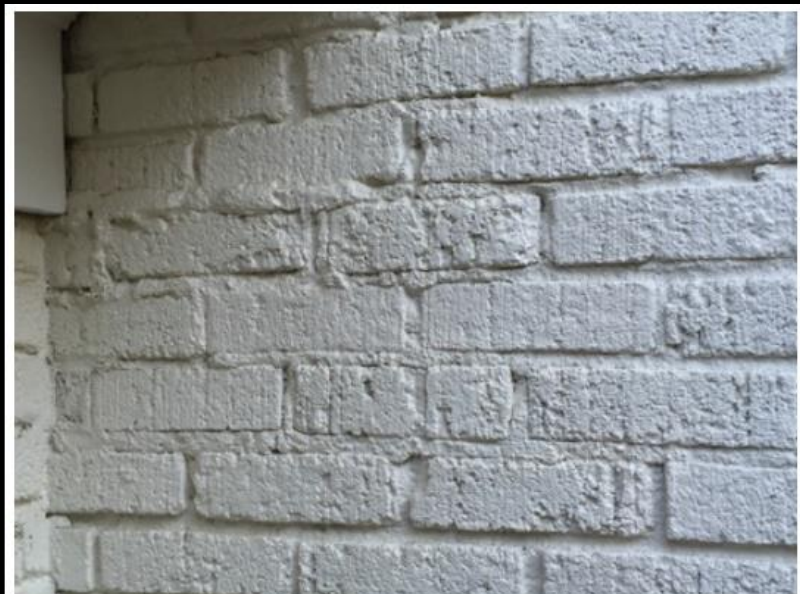
Same wall (higher up, w/o tape) of 1924 bldg. at SW side butt joint, facing Worthington. Unsightly-and problematic-overfilled and irregular mortar joints, inferior work all around.
