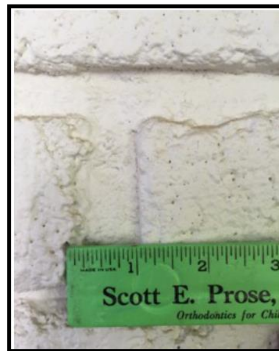
Mortar head joints in excess of one inch wide, common throughout all three sides of porch. (Industry standard is 3/8")
