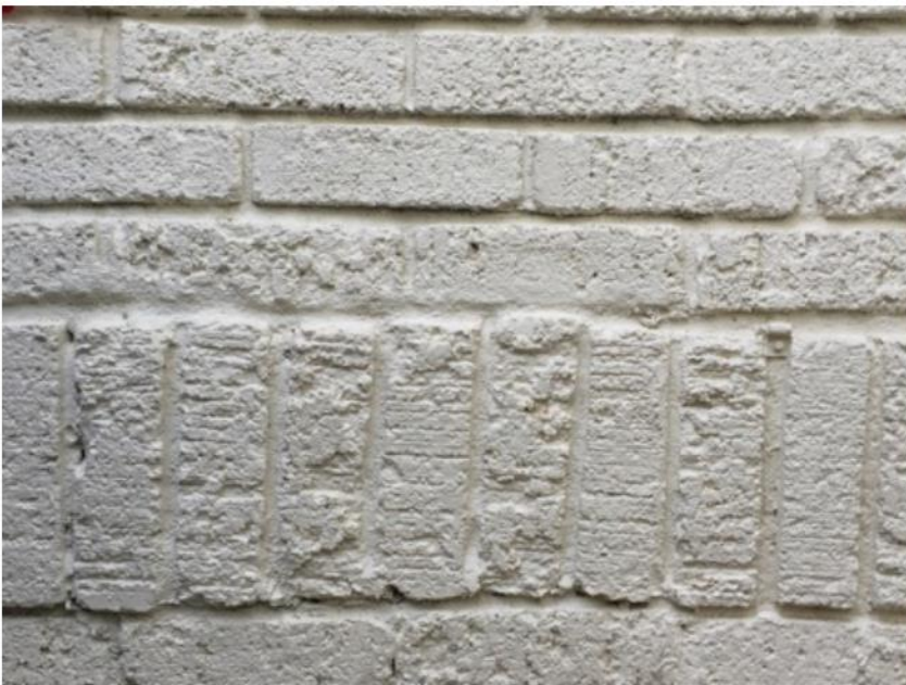
Crooked soldier course, NW wall of 2006 addition. Also note mortar overfill and drips
