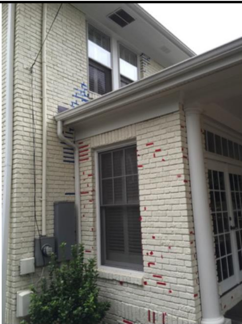
Northwest side of 2006 single story rear addition & original building. Settlement cracks around second floor windows carelessly repaired with blueish/gray mortar, instead of beige color used on rest of house. Tape below gutter illustrates uneven butt joint on this side of addition.
