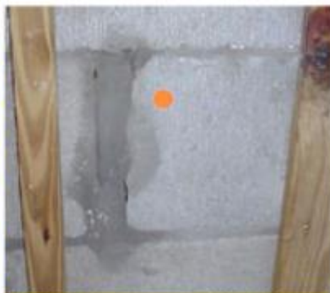
FIGURE 2: Improper mortar joint thickness.
