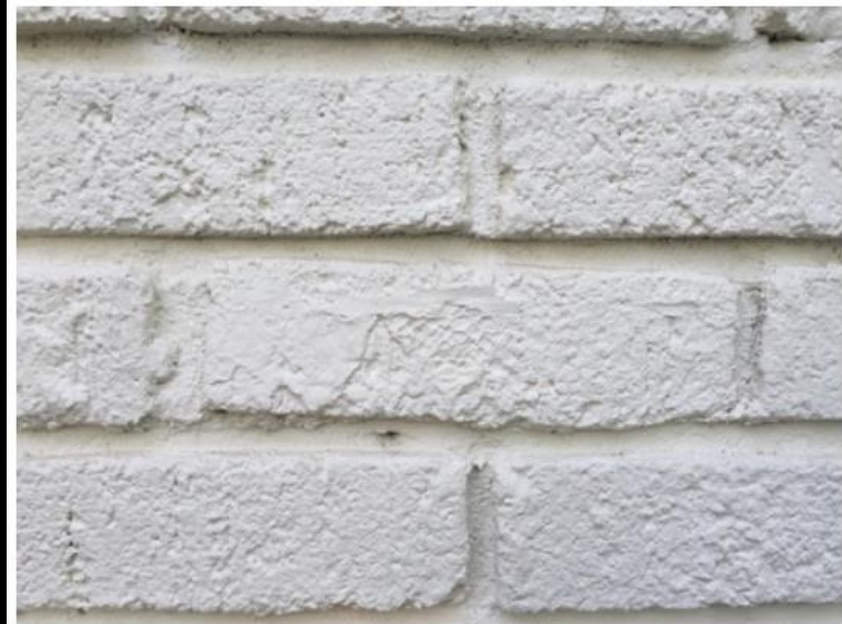
Crooked bricks, inconsistent mortar joint widths, shoddy mortar work- SW wall of 2006 addition, facing Worthington Ave.
