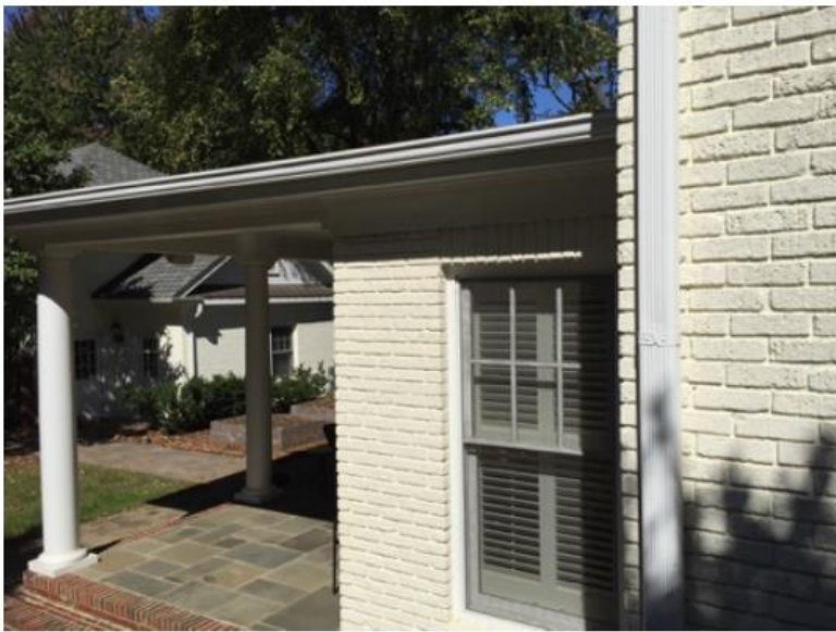
Inferior brick and mortar work on South wall of '06 addition (w/window) hidden by paint. Disparate elements of garage, addition and original house unified with neutral color.
