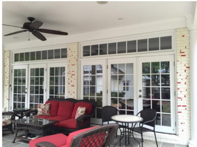
2006 rear addition. Red tape marks are a random sampling of the abundance of inferior masonry work, including: inconsistent mortar joint widths (from 1/4"-1 1/4"); broken bricks; crooked bricks; uneven course; overfilled mortar joints; excess mortar drips
