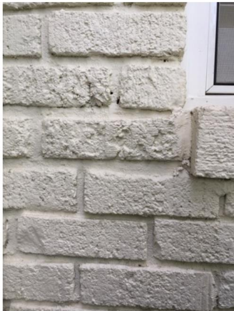
Northwest wall of 2006 addition, left side of window. Crookedly set bricks, broken bricks filled with mortar and inconsistent mortar joint widths.
