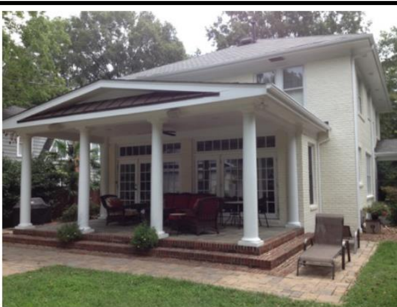
Poorly matched addition (porch) and repair work (2nd floor windows) hidden with paint, defects no longer visible from Worthington Ave.
