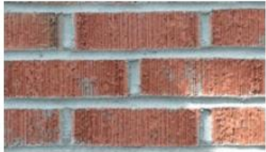
The bright red brick and gray mortar carelessly incorporated into the 2001 renovation came from the same batch of brick & mortar utilized in building the 2001 garage (left). Photo on the right is of the original 1924 brick & mortar.
