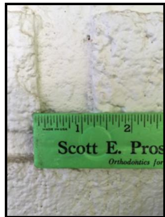
Inconsistent mortar joint widths; crooked and broken bricks; sloppy & excess mortar. Center wall of 2006 rear porch addition.
