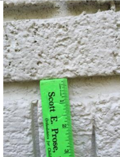
SW wall of 2006 rear addition. One of many head & bed mortar joints one inch wide. (industry standard is 3/8")
