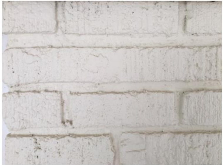
More inconsistent & sloppy mortar joints- right wall of 2006 addition
