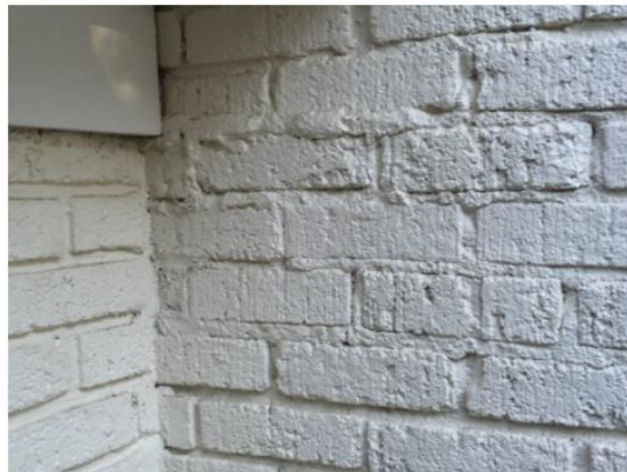
Despite being painted, this mismatched butt joint on the SW side , between the original house (right) and the 2006 addition (left), is clearly evident. Note once again the uneven rows of brick at the joint. The abundance of unsightly-and potentially damaging-mortar overfill on the upper right wall speaks for itself.
