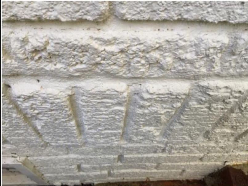
Top of crooked NW wall soldier course, protruding 1/4"-1/2" from rest of wall-exposing it to standing water.
