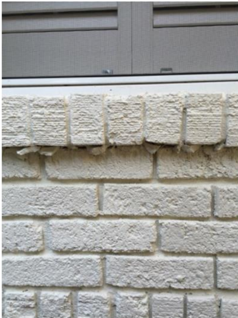
Crooked brick, irregular mortar joint spaces, sloppy mortar finish.
