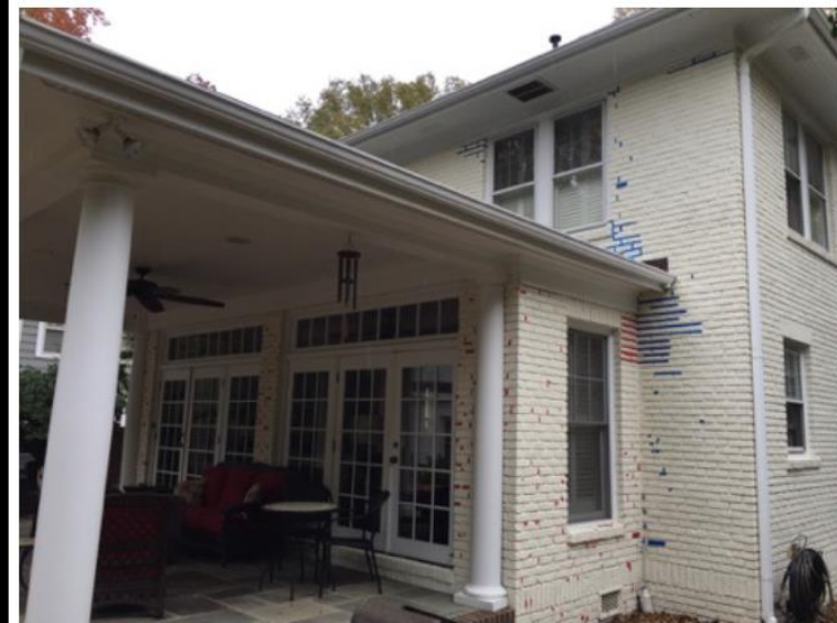
Southwest side of rear addition and original building, viewed from Worthington Ave walk. Tape below gutter illustrates a highly visible element of this poorly matched addition- the walls are uneven as much as 7/8" at the butt joint between old & new walls, and the mortar joints have been overfilled as much as 24" from the inside corner (blue tape)
