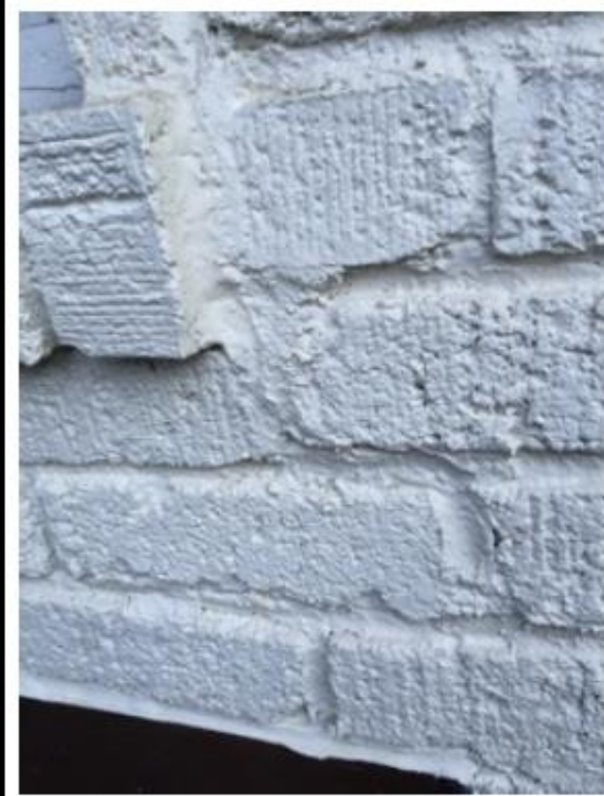
Poorly repaired settlement cracks around second floor rear window. The mortar color used was gray, despite the rest of the house having beige mortar. Probably done at the same time as 2001 renovation.
