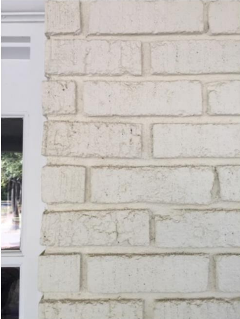
Uneven head & bed mortar joints, crooked & broken bricks-
