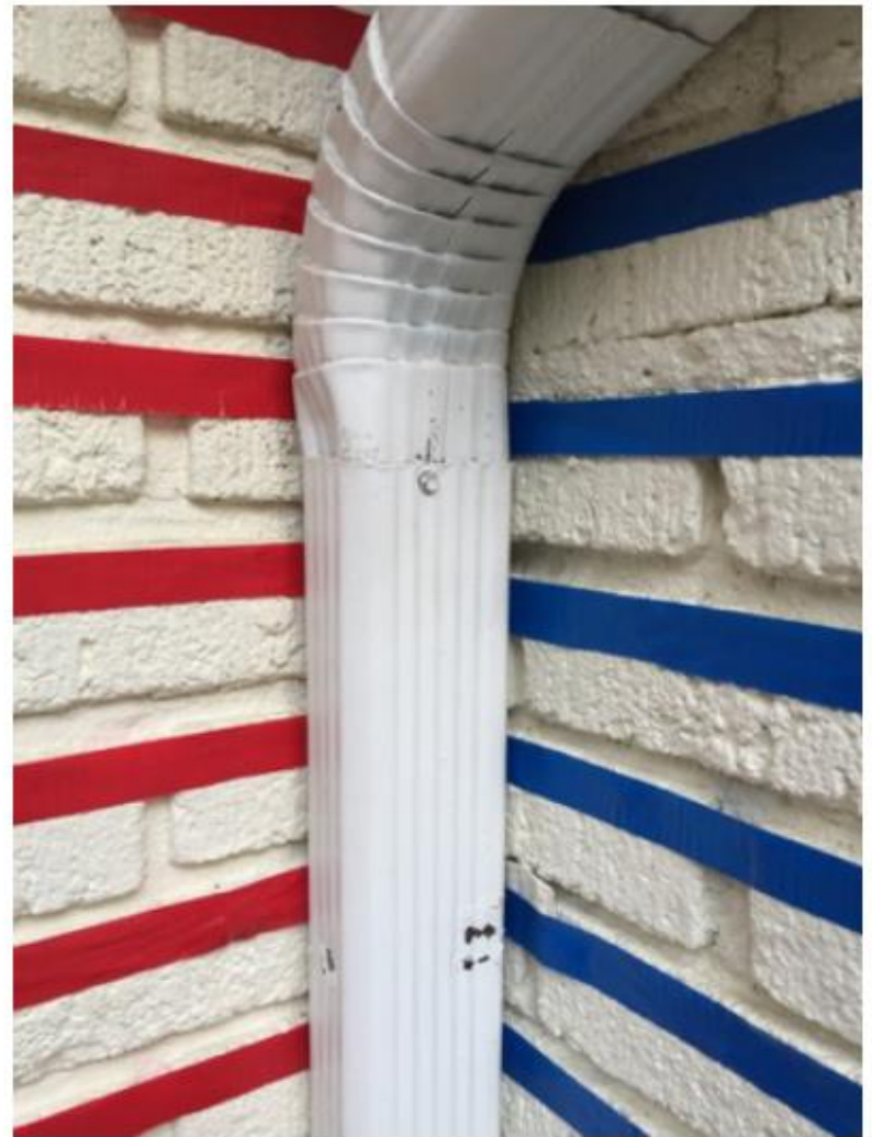
Greatly uneven brick courses at SW side butt joint facing Worthington Ave. of 2006 addition (left) and 1924 original structure (right), some as much as 7/8" Also note irregular mortar joints, as well as overfilled joints at top right.
