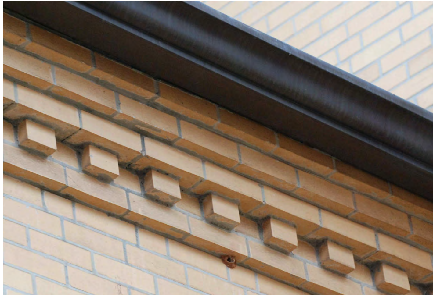
P1 EXISTING BRICK DETAIL AT WALL EAVE
