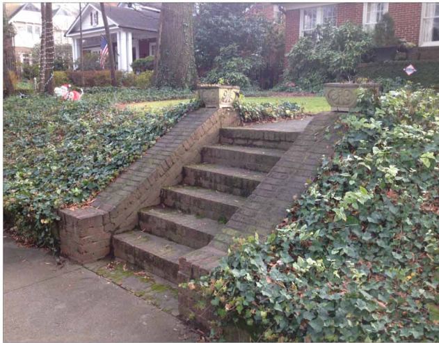
C EXISTING BRICK CHEEK WALLS AT 712 MT VERNON AVE NOT TO SCALE
