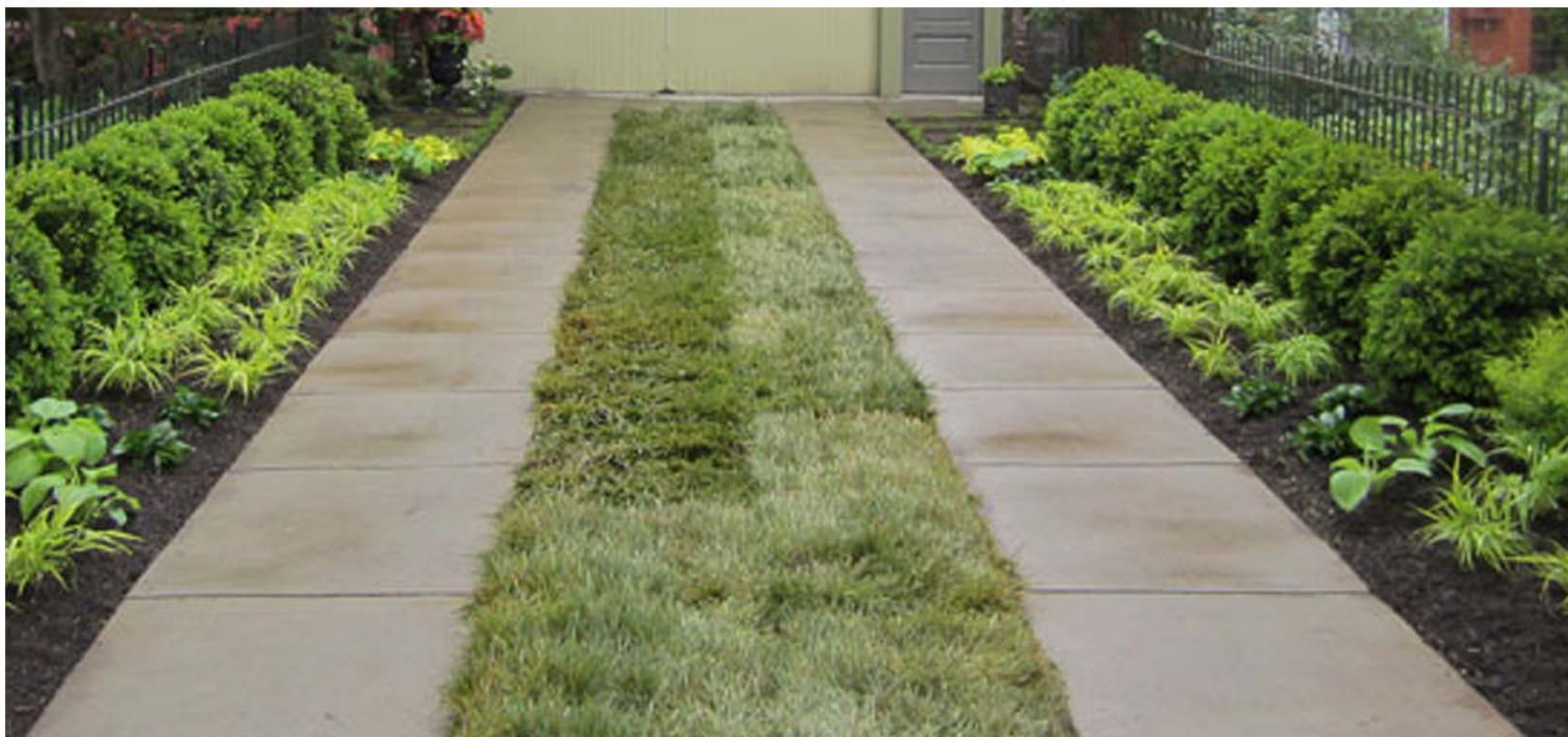
CONCRETE CARRIAGE DRIVE WITH CONCRETE PAVER MEDIAN
