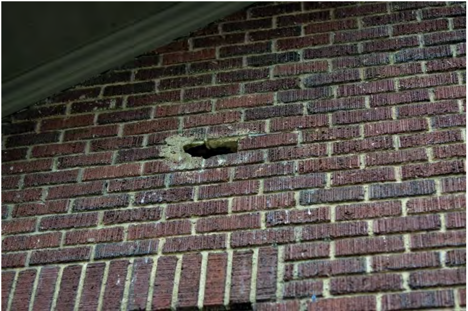
upper left side of house- hole in brick with clumped mortar in need of repair
