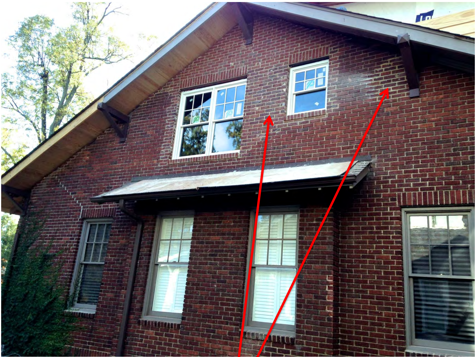
right side of house, post interior renovation-even with the closest match in brick the repairs are obvious
