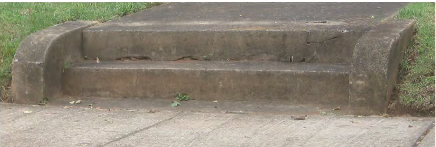
CONCRETE CHEEKWALLS
