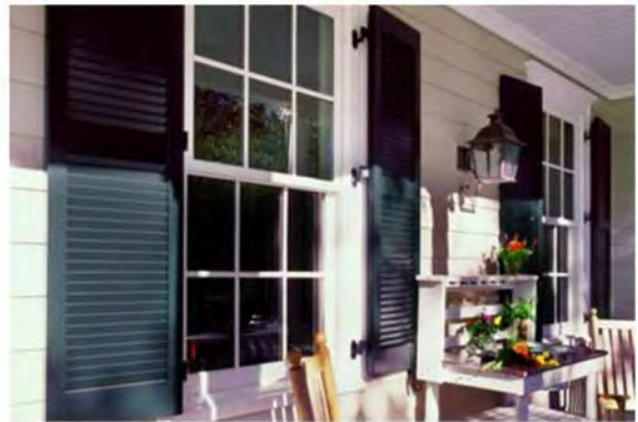
WINDOWS: PAINTED WOOD INSULATED WINDOWS MULLIONS ON EXTERIOR & INTERIOR 6 LITES OVER 0
