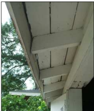
EAVE DETAIL WITH EXPOSED RAFTER TAILS
