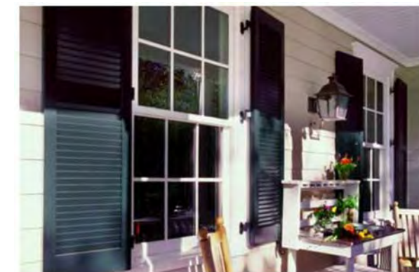
WINDOWS: WINDSOR LEGENDS SERIES PAINTED CELLULAR PVC MULLIONS ON EXTERIOR & INTERIOR 6 LITES OVER 0
